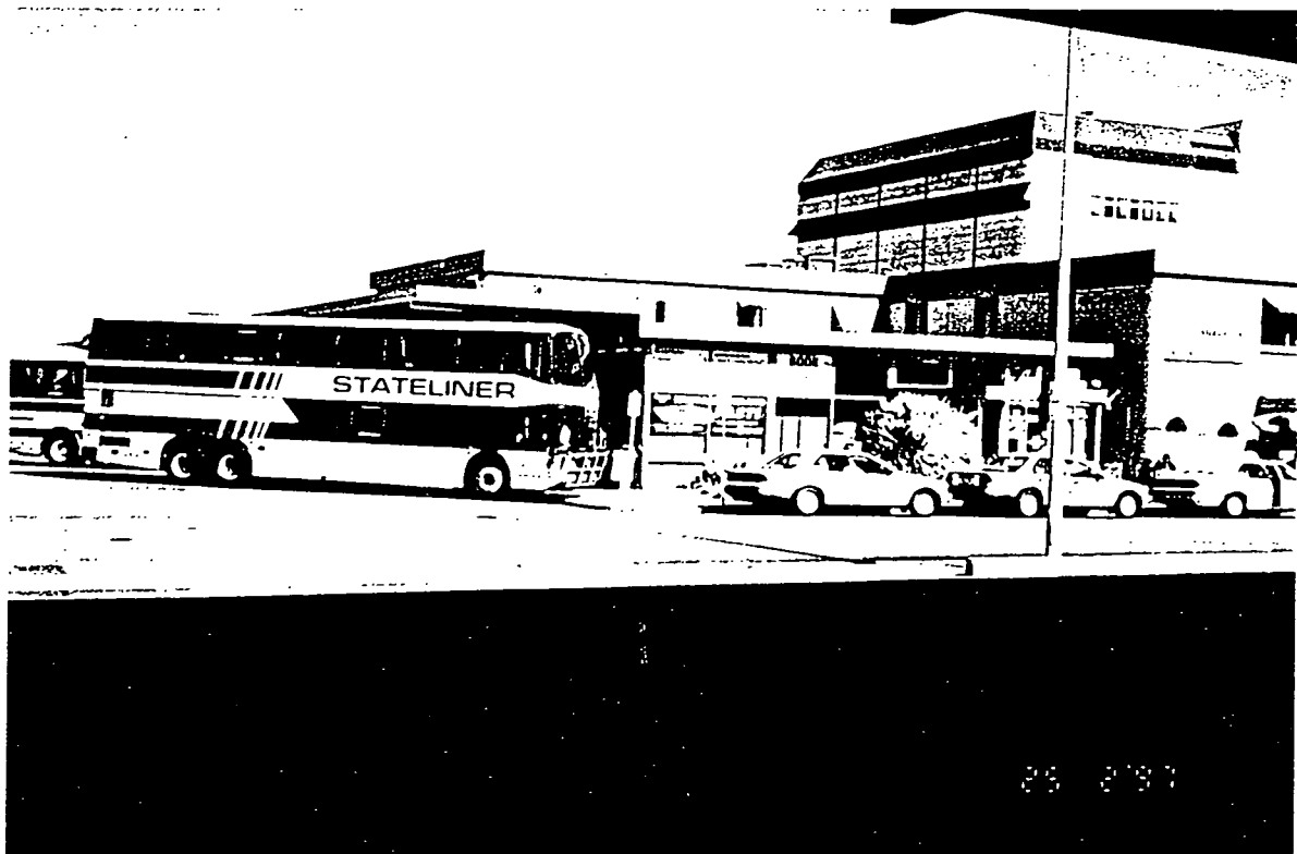
Photo 4: The Premier Stateline passenger terminal, and attached canopy for bus parking (looking west across Bowen Street).
