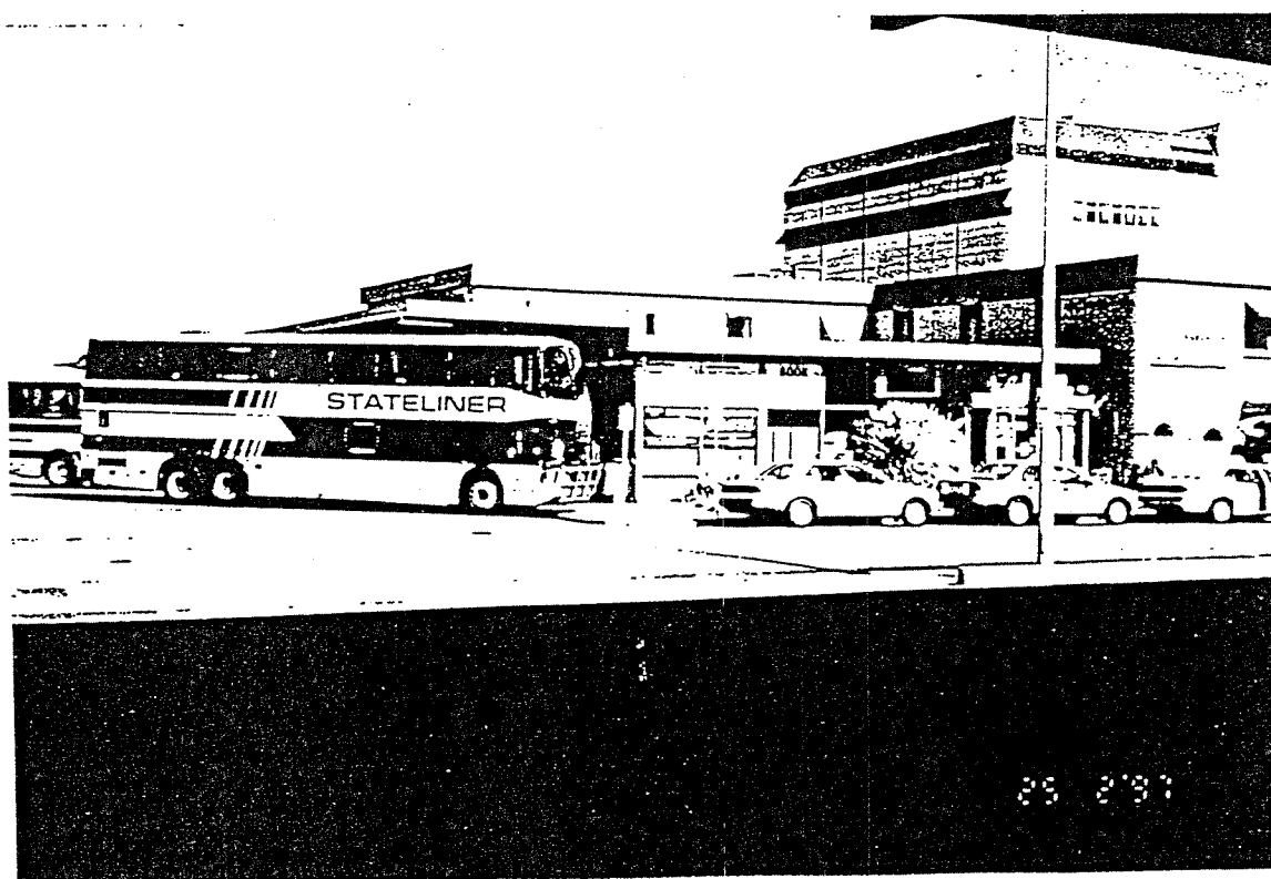
Photo 4: The Premier Stateline passenger terminal, and attached canopy for bus parking (looking west across Bowen Street).
