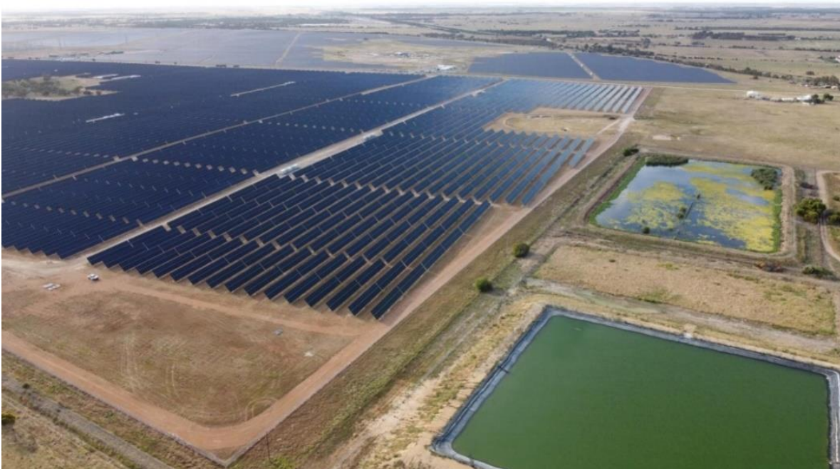
Figure 12a: Example solar modules (Tailem Bend Solar, Vena Energy)
