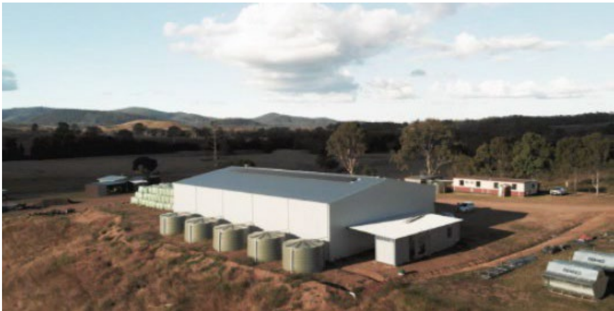
Figure 3-13 Example of a typical operations and maintenance building
