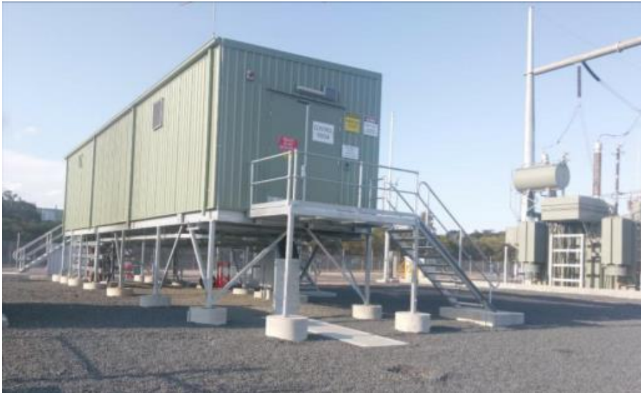
Figure 12c: Example switchroom
