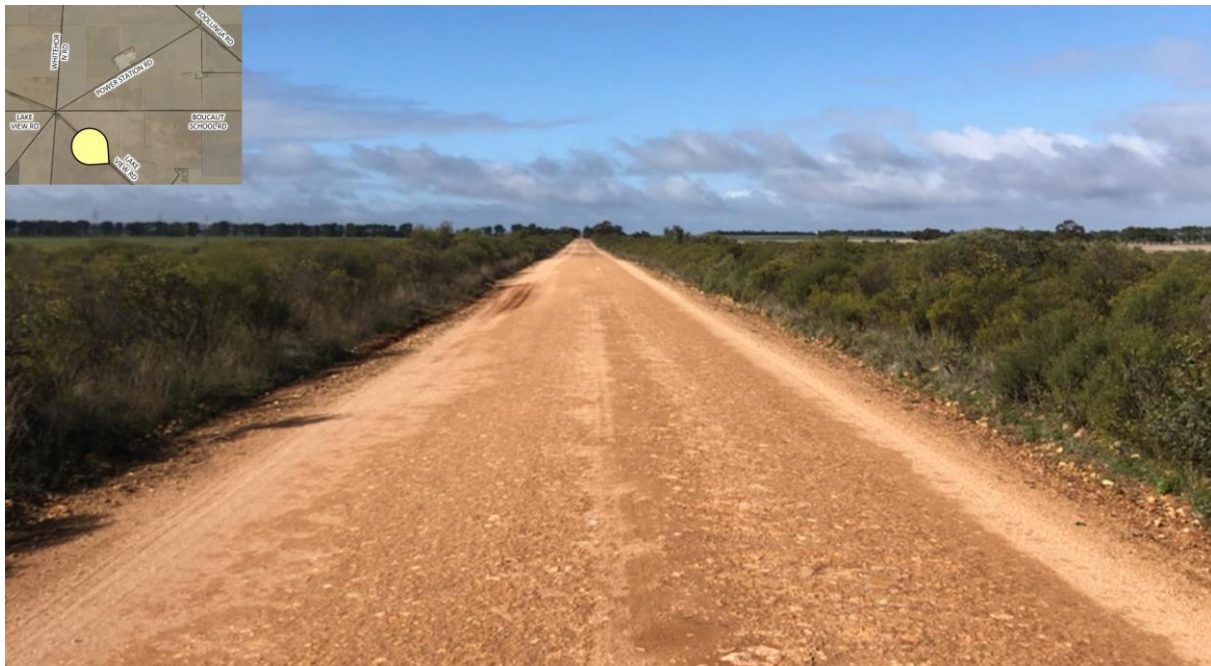
Figure 2.5: Lake View Road (looking south-east)
