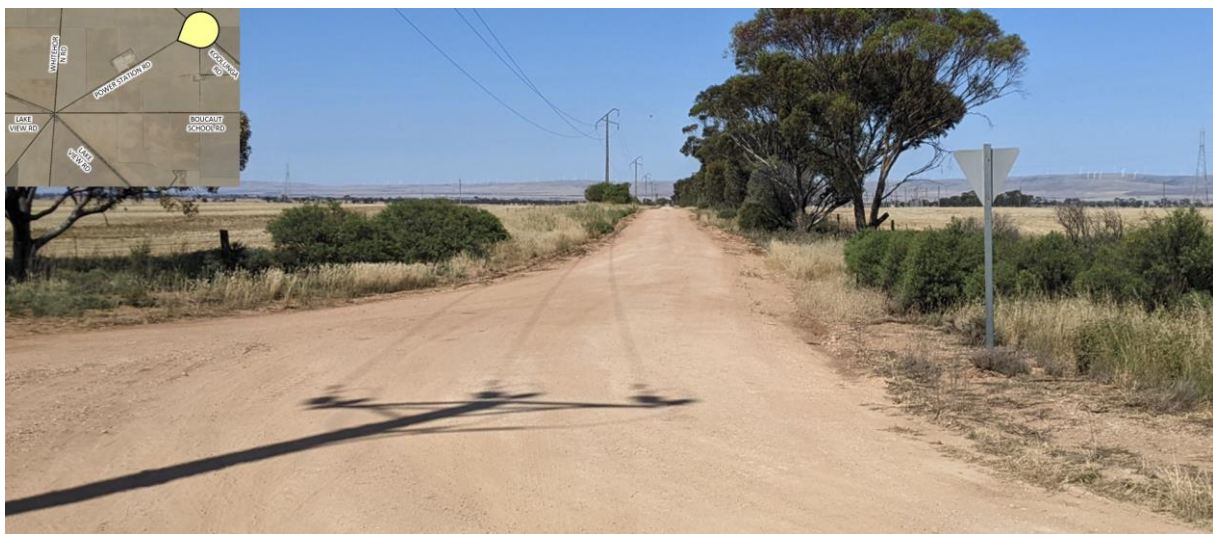
Figure 6.2: Power Station Road (looking south-west from Koolunga Road)
