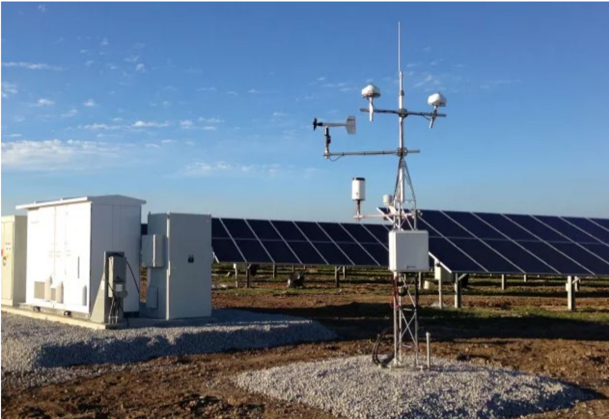
Figure 3-10 Example of weather station at solar farm (source: Campbell Scientific)
