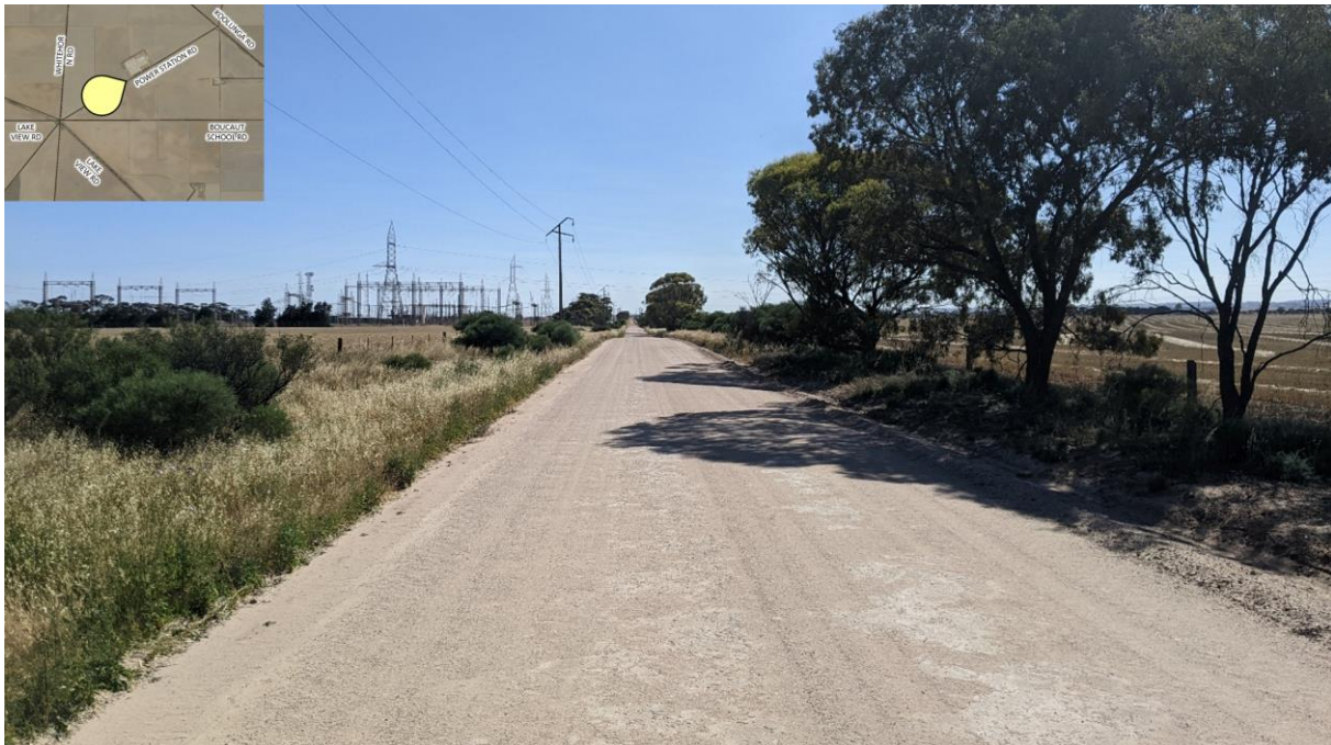
Figure 2.2: Power Station Road (looking north-east towards Substation)
