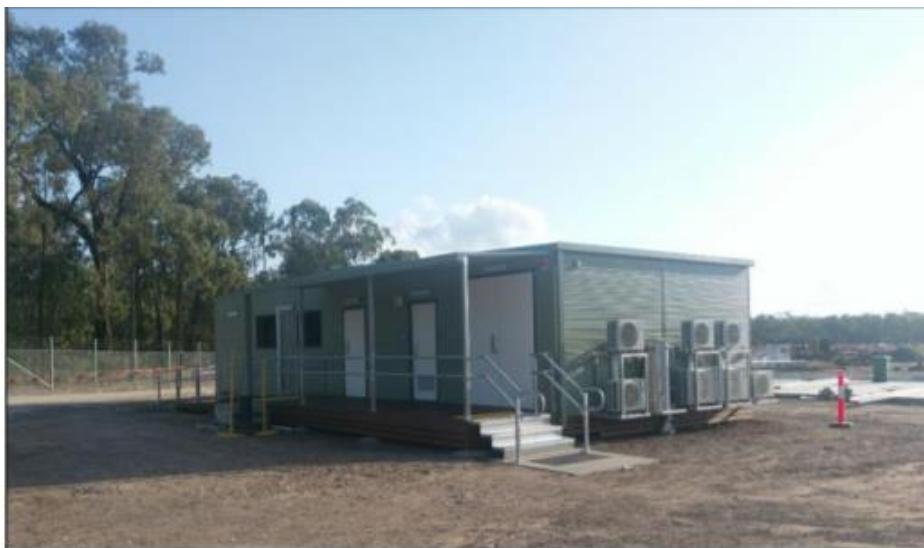
Figure 12d: Example control room
