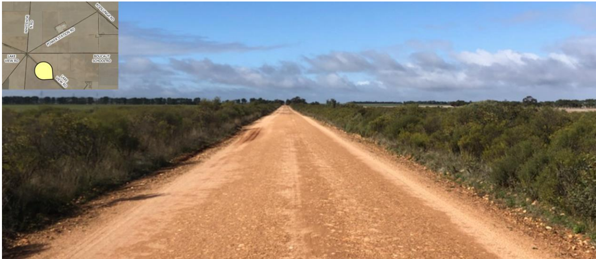
Figure 6.4: Lake View Road (looking south-east)
