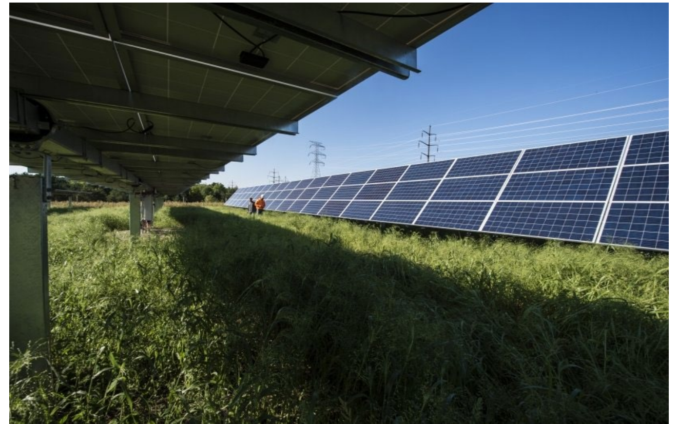
Image 3: Example of an array Pv solar panels
