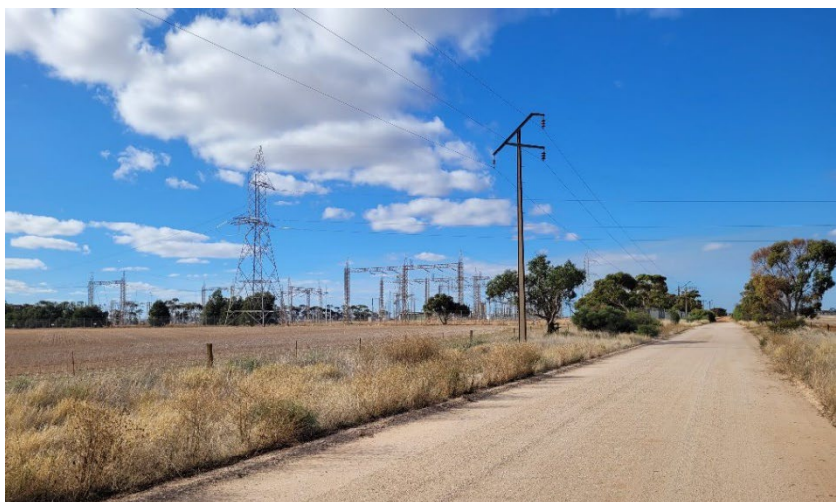
Figure 1-5 Existing Brinkworth substation viewed from Power Station Road
