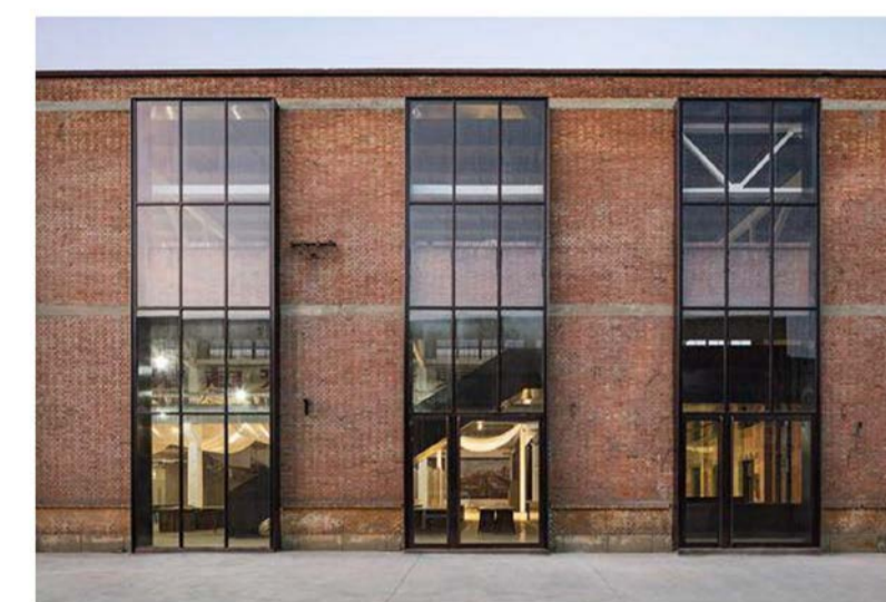
ANCILLARY RETAIL FACADE DESIGN IDEA - BRICKSNAP PRECAST & ALUMINIUM FRAME GLAZING SYSTEM
