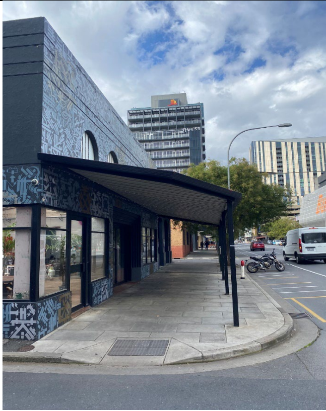
Photo 3.7: Front of site looking east
