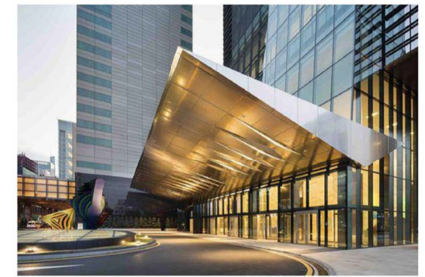
FEATURE METAL CLAD CANOPY
