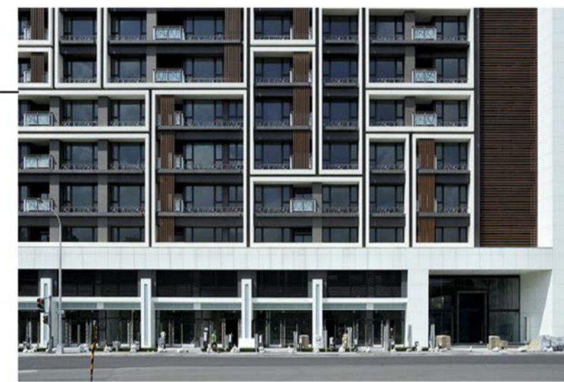
APARTMENT FACADE DESIGN IDEA - PRECAST CONCRETE PANEL & LIGHT WEIGHT MATERIAL & GLASS BALUSTRADES
