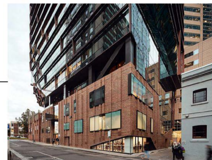
ANCILLARY RETAIL FACADE DESIGN IDEA - BRICKSNAP PRECAST & ALUMINIUM FRAME GLAZING SYSTEM
