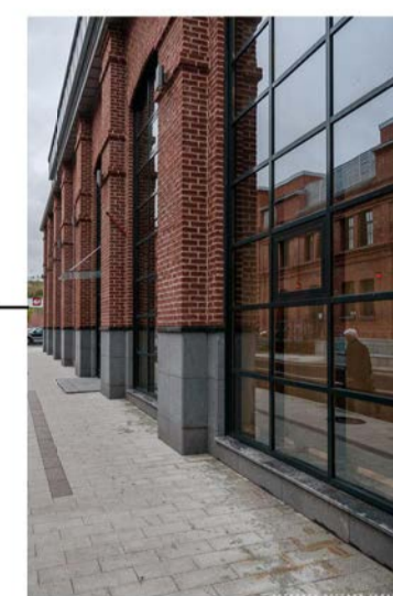
ANCILLARY RETAIL FACADE DESIGN IDEA - BRICKSNAP PRECAST & ALUMINIUM FRAME GLAZING SYSTEM
