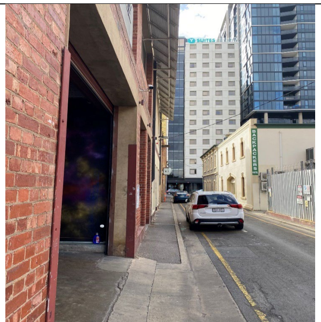
Photo 3.2: Eastern side looking north
