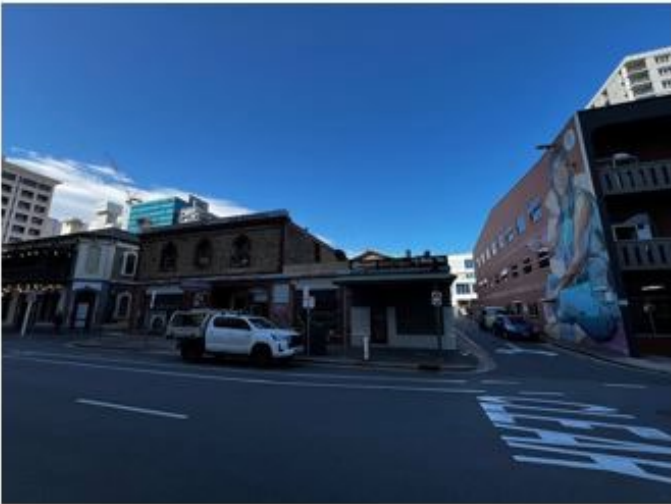
Photo 9: Waymouth Street facing south
