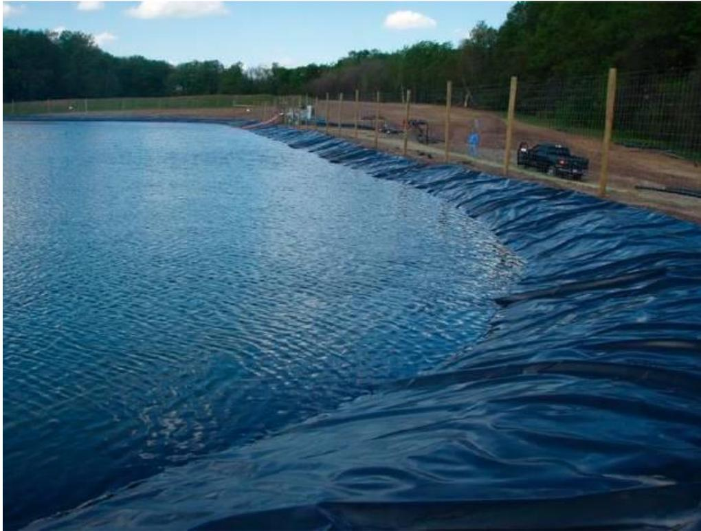
**Figure 39: Example of lined retention basin** (Appendix C3 Figure 5.5)
