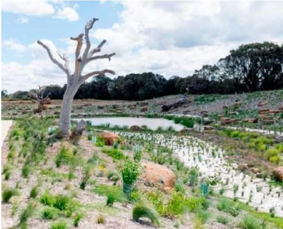
**Figure 37: Example of a vegetated ephemeral wetland basin with inlet swale** (Appendix C3 Figure 5.1)
