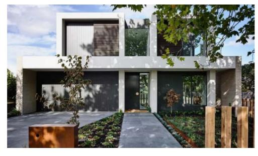
2. Charcoal steel cladding areas, similar to corrugated roofs in the area 3. WHITE HEBEL, TO TIE IN WITH WHITE CONCRETE TO MIXED USE BUILDING.
