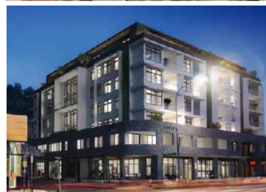
248-252 UNLEY RD HYDE PARK PLACE 7 STOREYS BUILT
