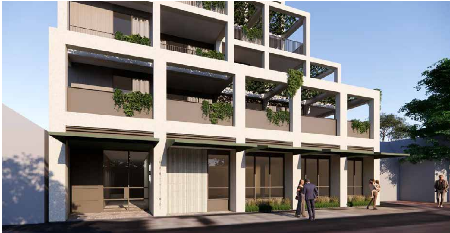
EASTERN FACADE VIEW FROM UNLEY ROAD
