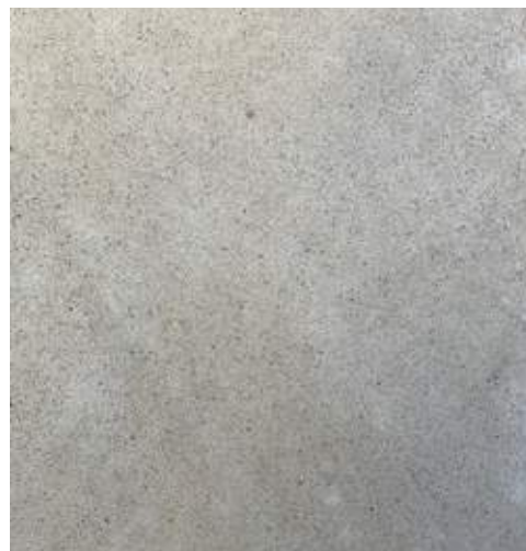
↑ INSITU CONCRETE (CARPARK)
