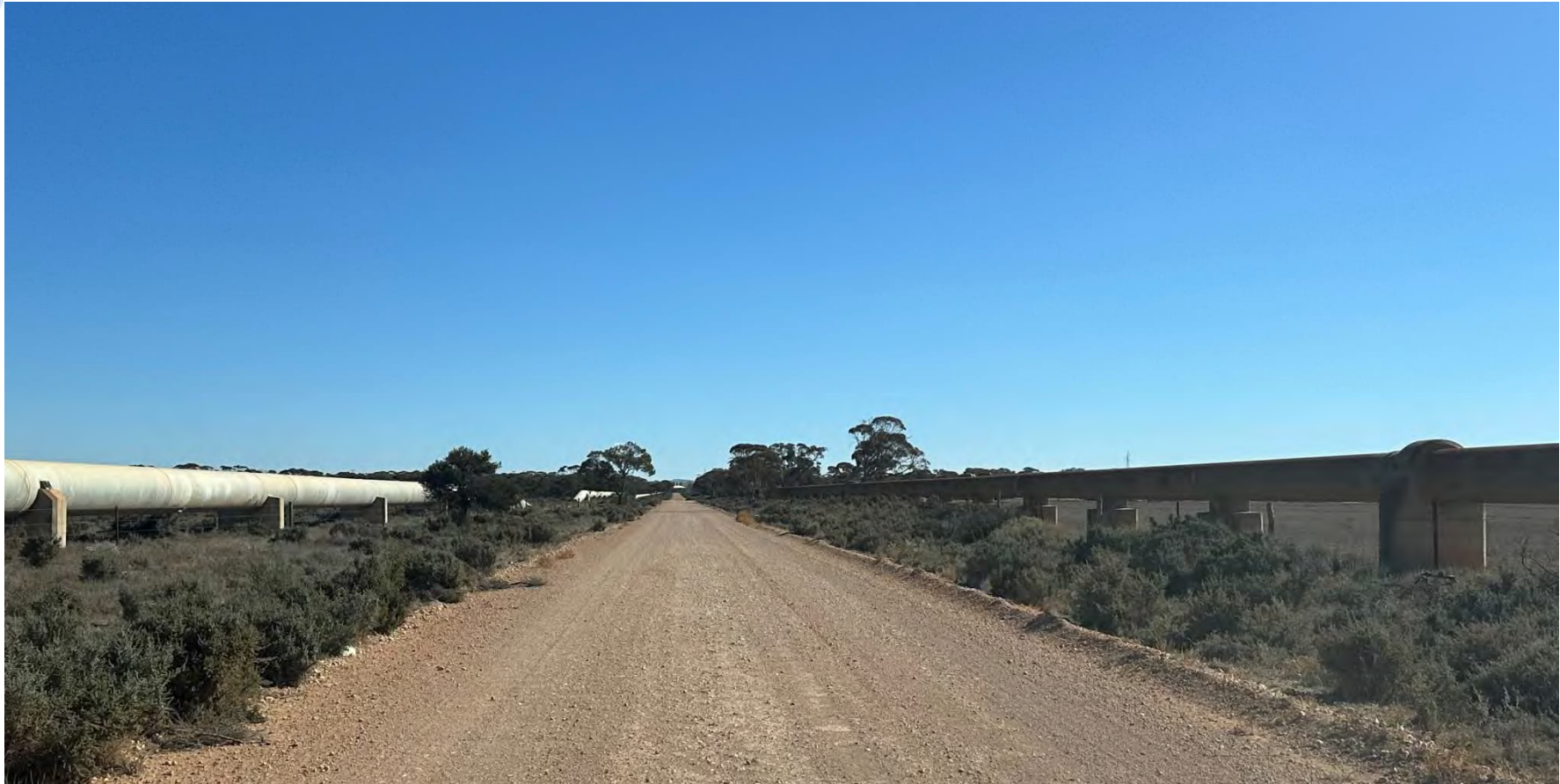
Figure 5-20: View along Pipeline Road (Looking West)
