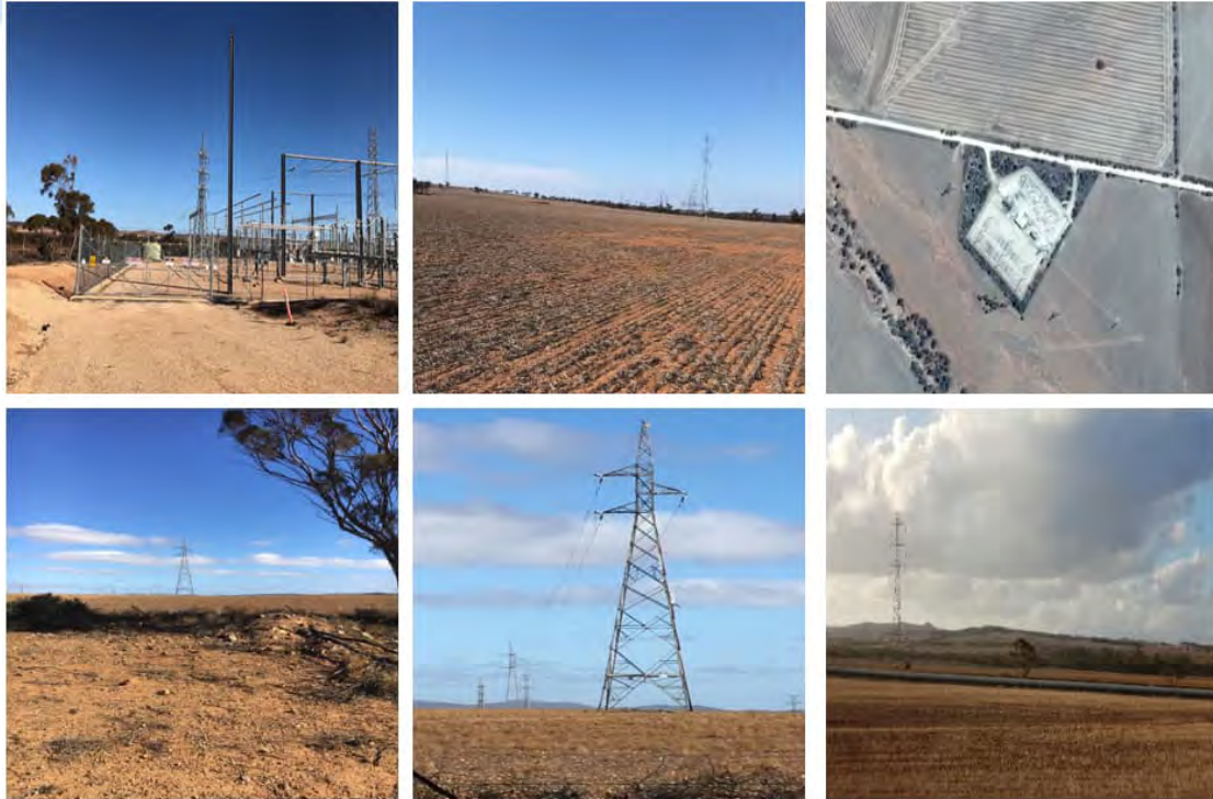
Figure 2-6: Existing Electrical Infrastructure Around the Project Area
