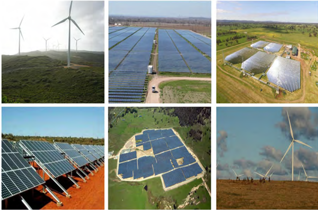
Figure 2-3: Existing Renewable Infrastructure in Australia
