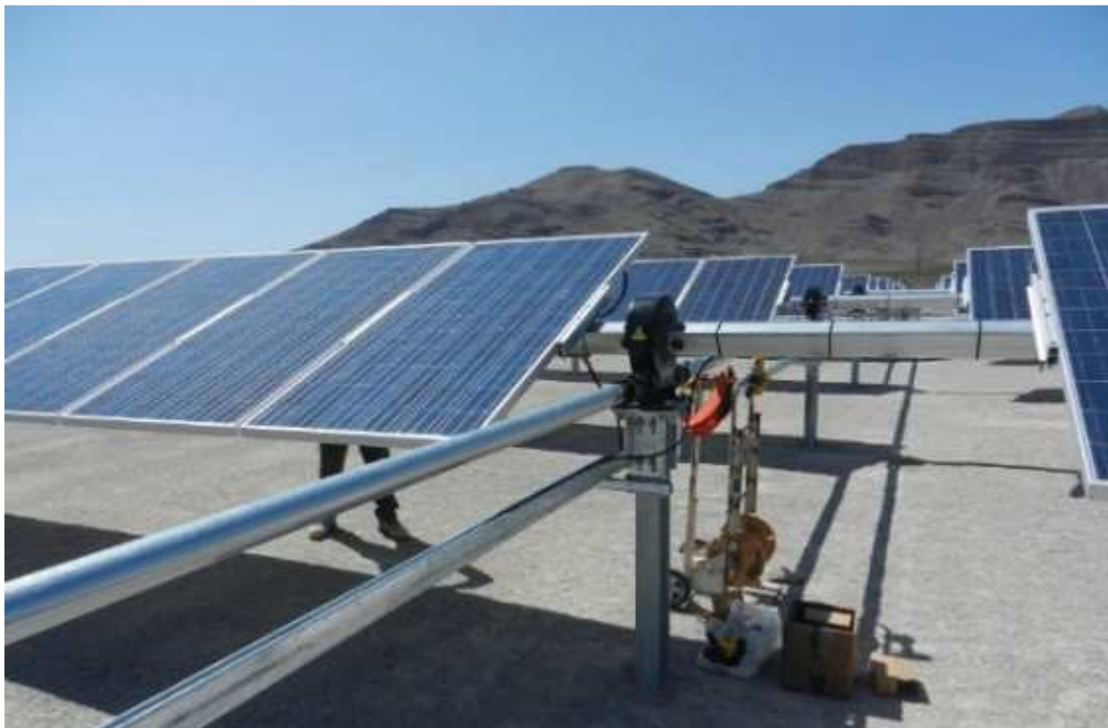
Plate 2-12: Typical photovoltaic panel with a single axis tracking system (Source: SNC-Lavalin)
