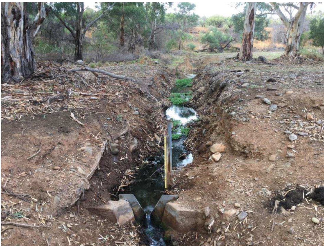
Figure 6. Spring flow and gauging weir below Baroota Reservoir wall. (photo: J Carter)
