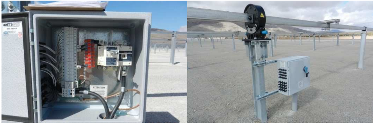
Plate 2-15: Typical single axis tracking racking system and combiner box (Source: SNC-Lavalin)
