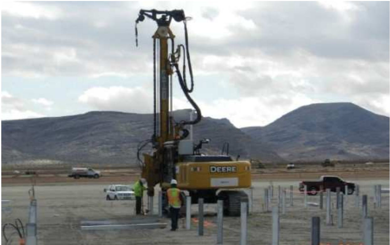
Plate 2-13: Typical piling operation to install mounting poles (Source: SNC-Lavalin)
