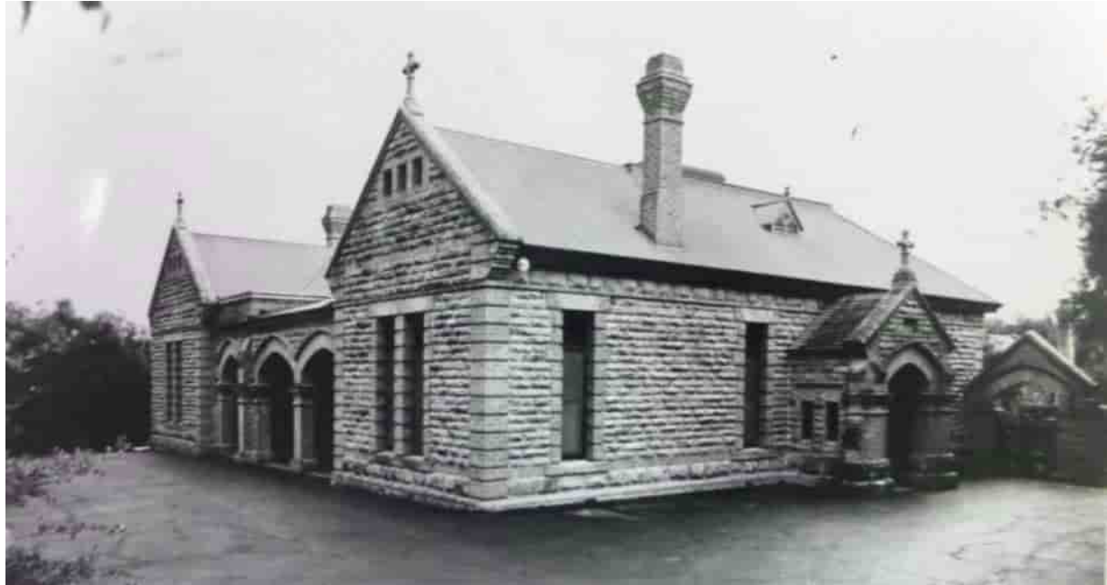
Figure 3: Early photo (n.d. – c.1900) of house as first constructed, from the south-east. The front (south) elevation/entry was accessed through the arcaded verandah and the east elevation was later substantially changed with the erection of the 1957 chapel
