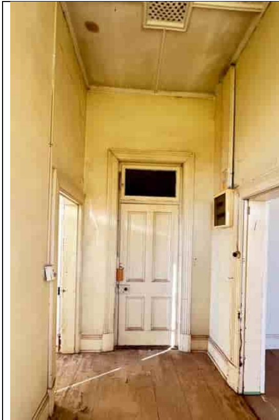
Room 13. Staff Room – to be combined with Room 12 into a fine dining room
