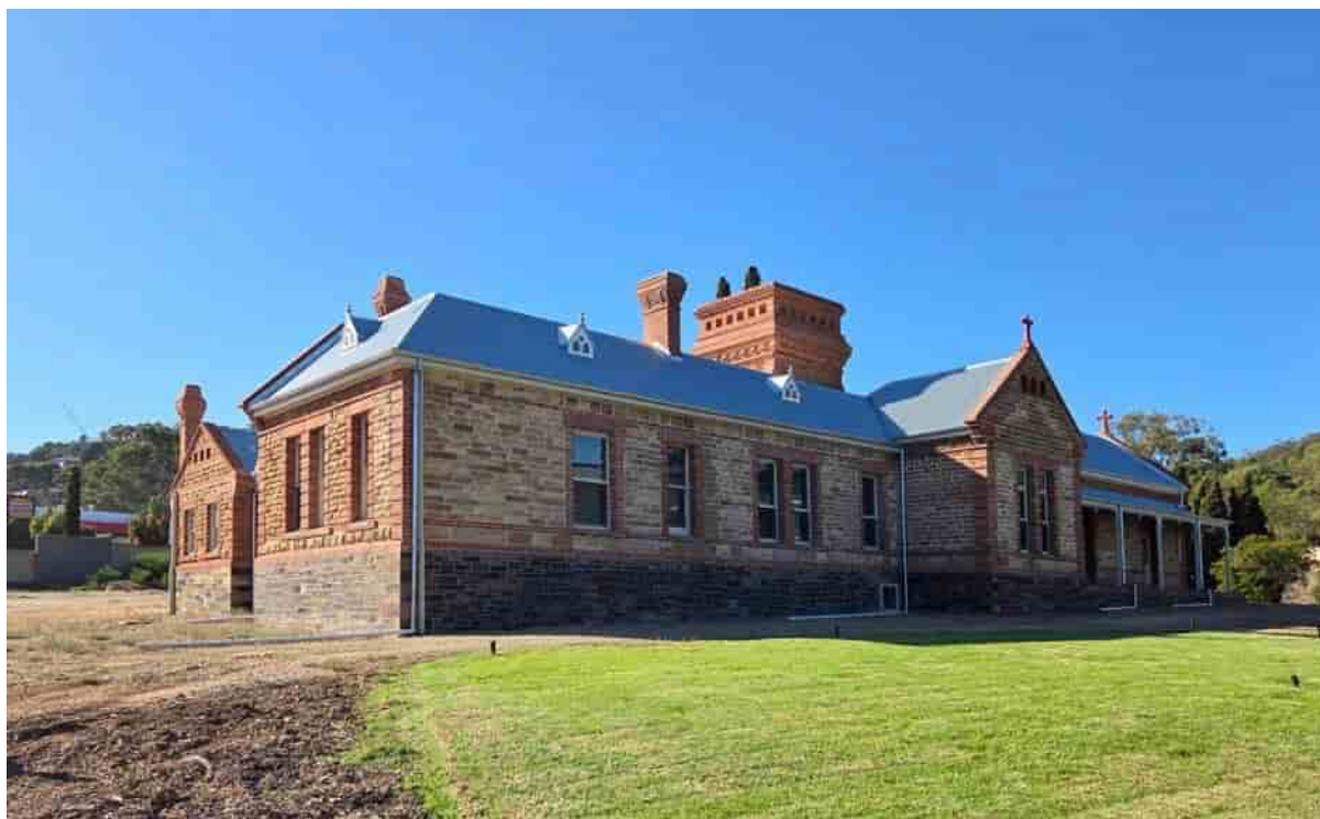
Figure 8: North-west view, 2025 Source: Hosking Willis Architecture
