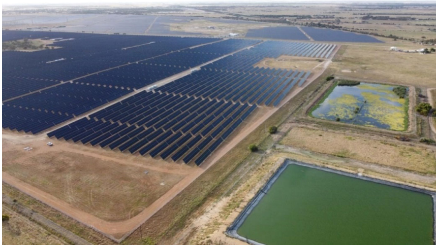
Figure 12a: Example solar modules (Taillem Bend Solar, Vena Energy)
