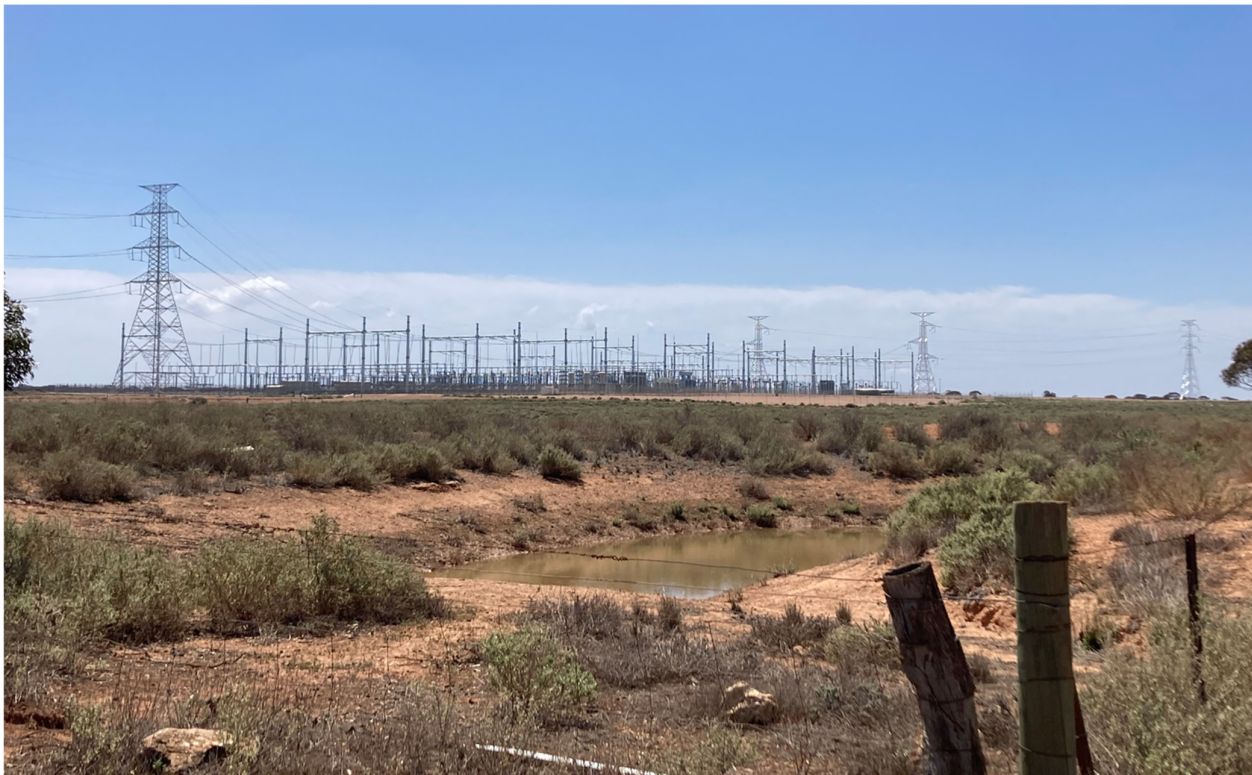
Figure 10: Bunday Substation – photo taken 23 October 2024
