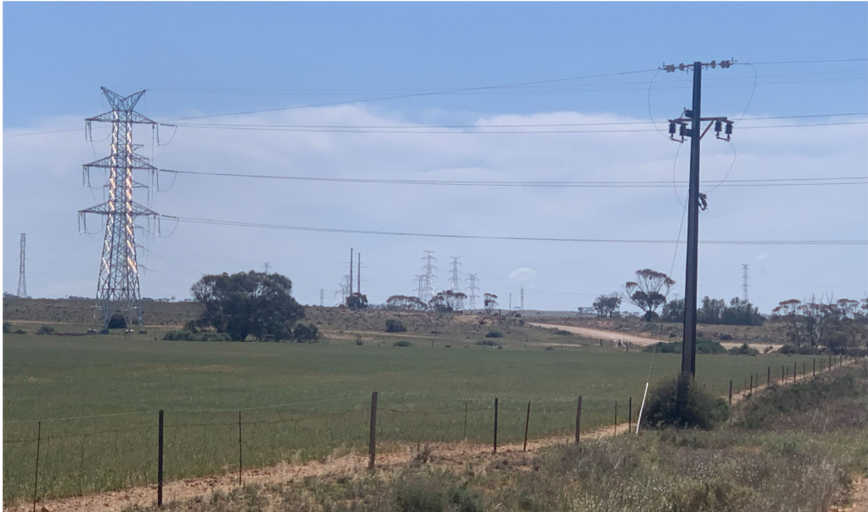
Figure 9: Existing electricity transmission infrastructure – photo taken 23 October 2024
