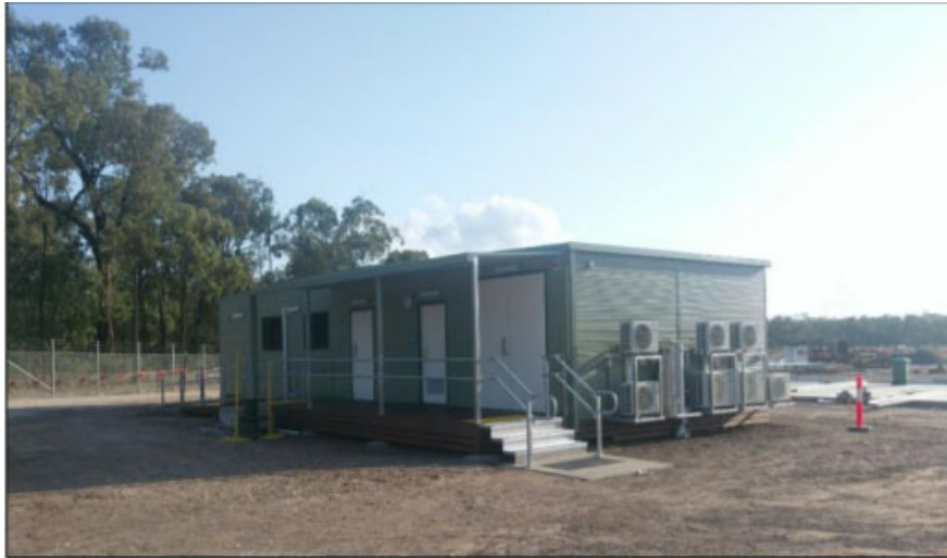
Figure 12d: Example control room
