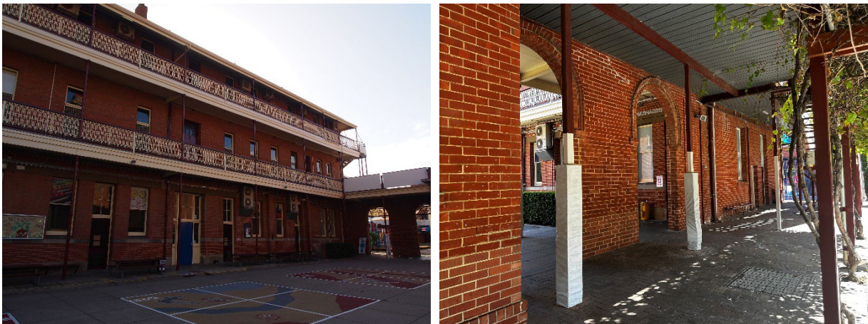
Figure 11: Dunlevie Building external views of southern wall showing external balconies and external stair
