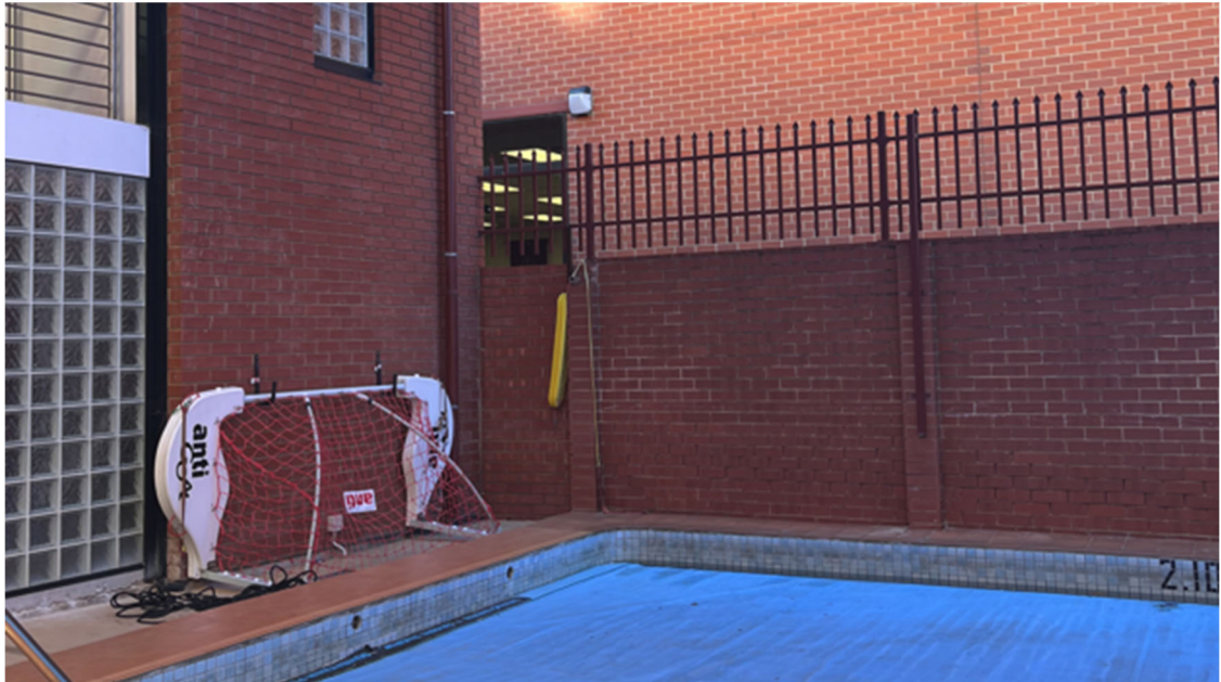
Photograph 1: Existing boundary wall between the pool enclosure and Archdiocese Centre.
