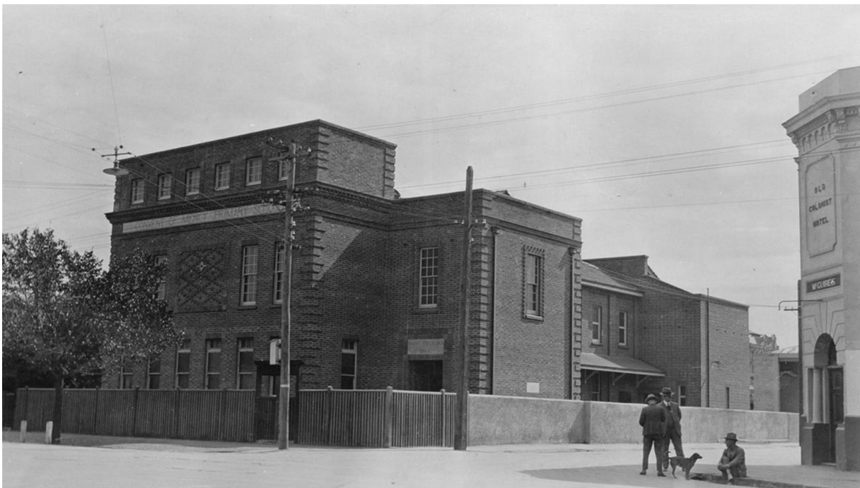
Figure 39: St Cecilia's Hall and Parish School – two storey building with a one three storey section constructed of brick and featuring a motif on the wall with a geometric pattern including a cross (State Library of South Australia, 1926, B-13408)
