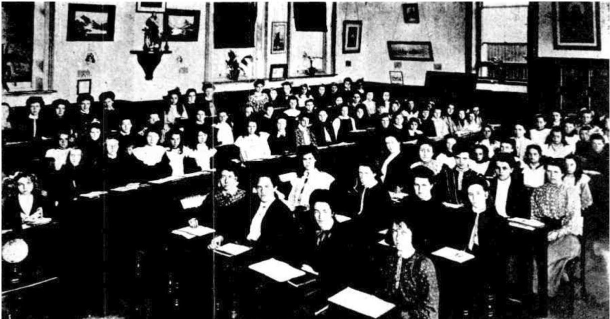
Figure 28: Interior of new school room, Angas Street (St Aloysius College,, circa 1906)
