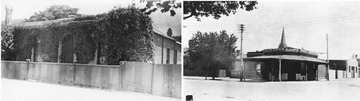
Figure 37 Angas Street cottage, demolished in 1923 (State Library of South Australia, 1922, B-1108)
