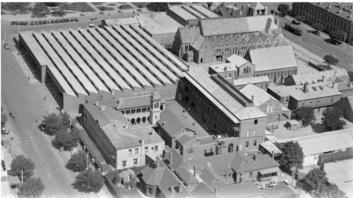
Figure 43: Aerial view of the Convent of Mercy, Cunningham Memorial Chapel and Dunlevie Building, with the MTT tram barn, St Francis Xavier's Cathedral, St Xavier's School Hall, and House of Mercy Building in the background. The Barr Smith House can be seen in the foreground (State Library of South Australia, 1930, BRG-397-2-45-9 (partial))
