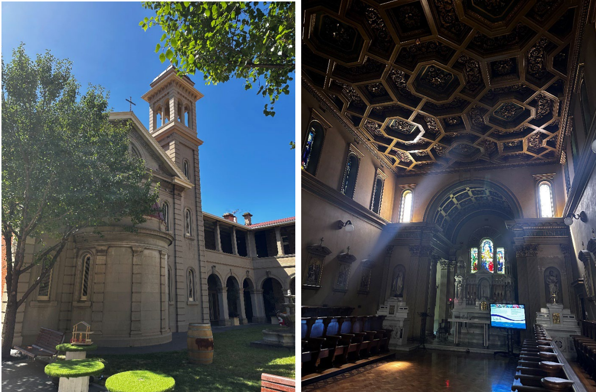
Figure 07 and 08: Cunningham Memorial Chapel, external and internal views
