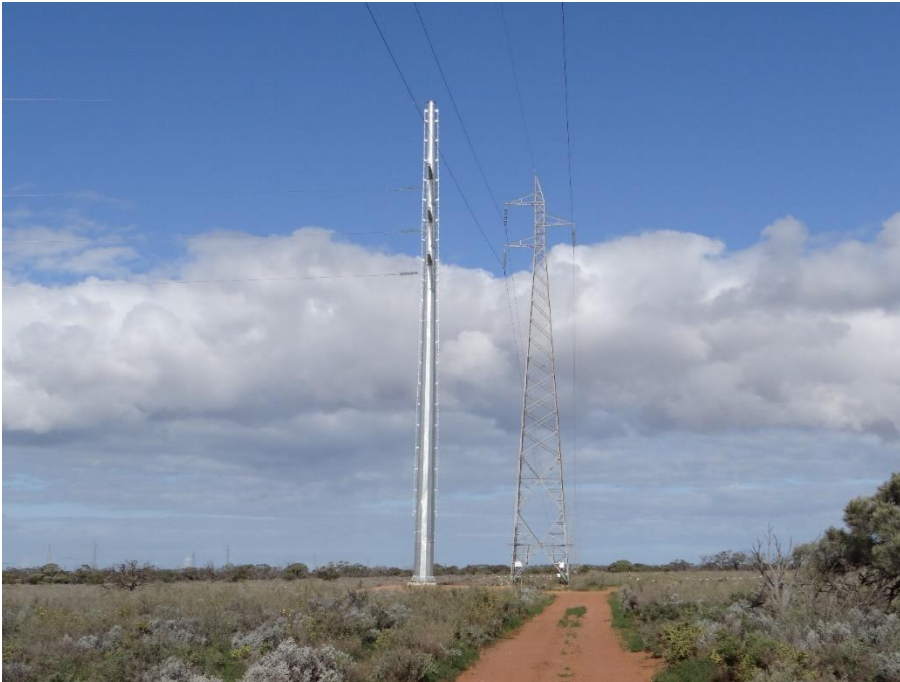
Plate 2 – Example 132 kV pole and tower (Source: ElectraNet)
