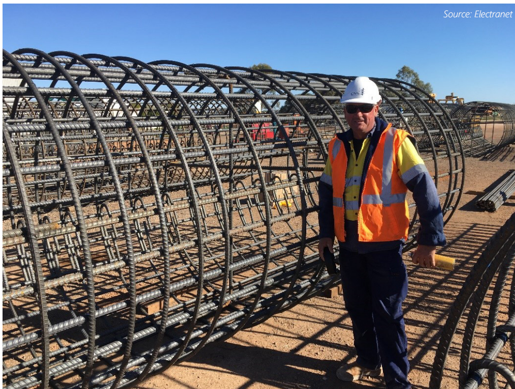
Plate 5.4: Typical Pole Footing
