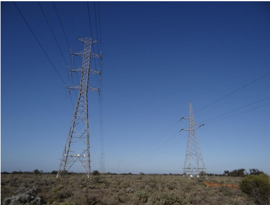
Plate 1 – Lattice Towers (132 kV on right, 275 kV on left) (Source: ElectraNet)
