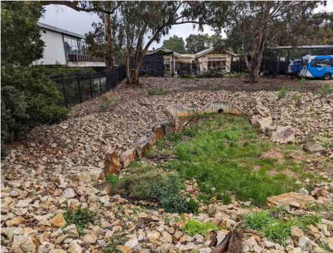
Figure 5: Existing Detention Basin
