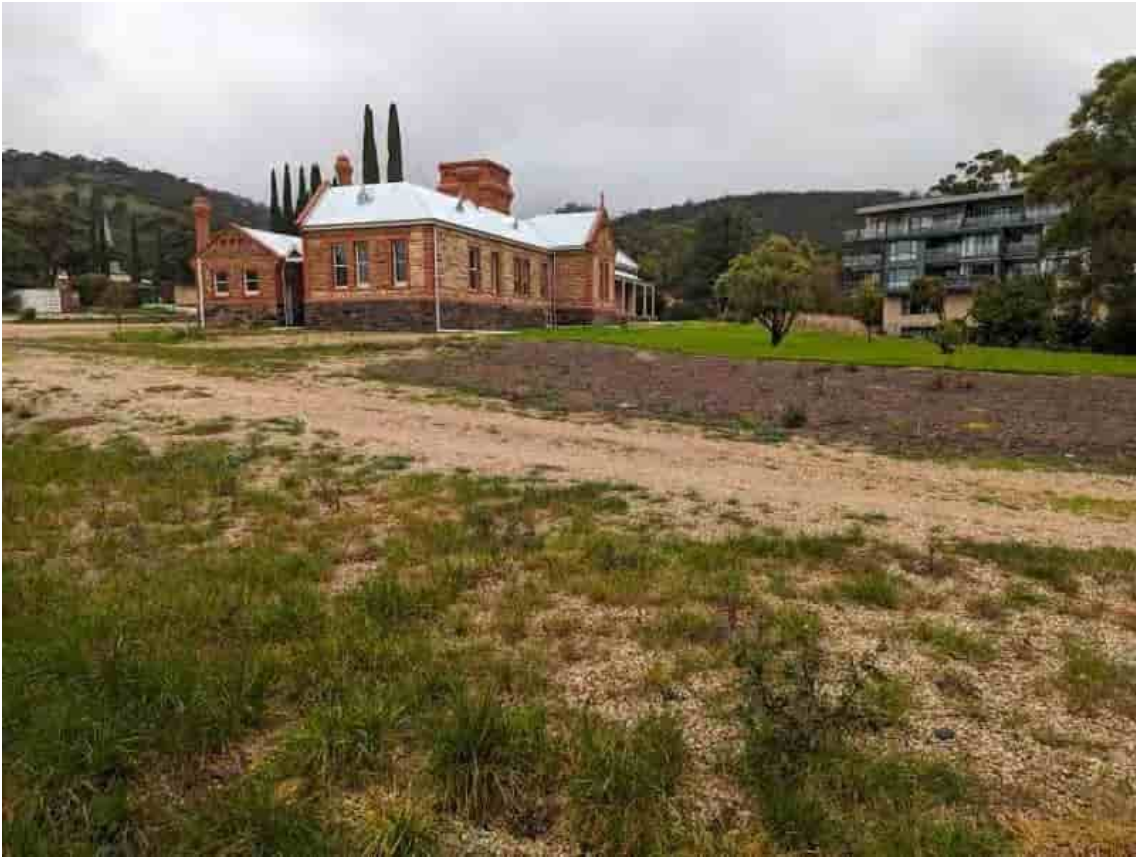
Figure 2: Existing Arch Bishop's Residence Looking South-West from Northern Boundary
