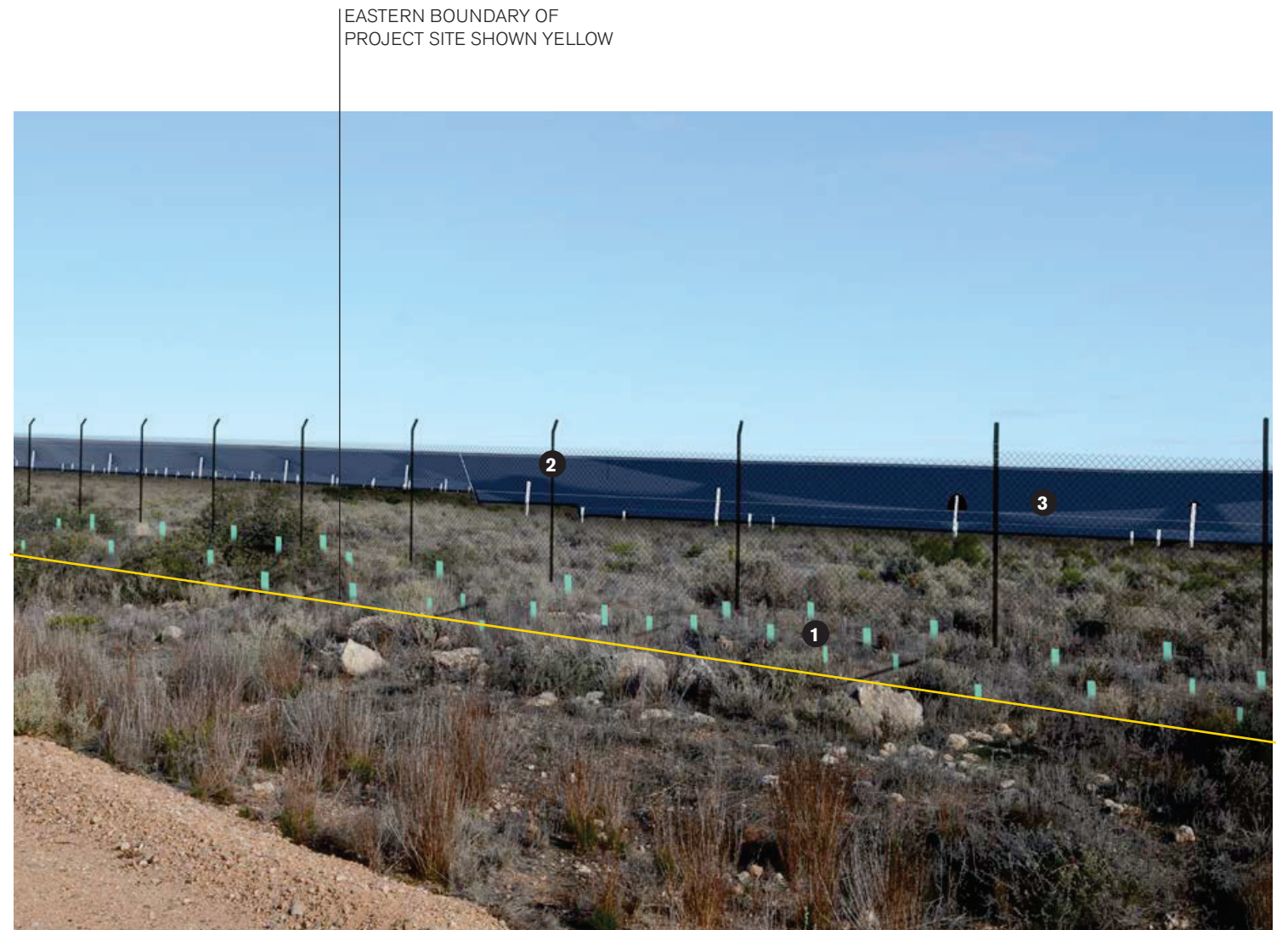
VIEWPOINT 09 - COMPLETION OF SOLAR FARM & FENCE
