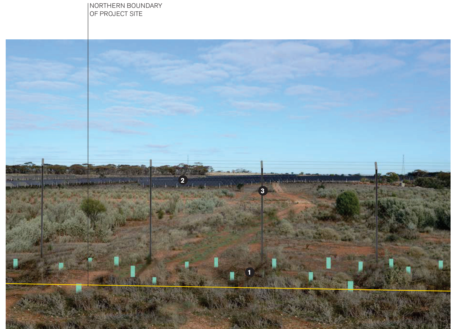
VIEWPOINT 06 - COMPLETION OF SOLAR FARM & FENCE
