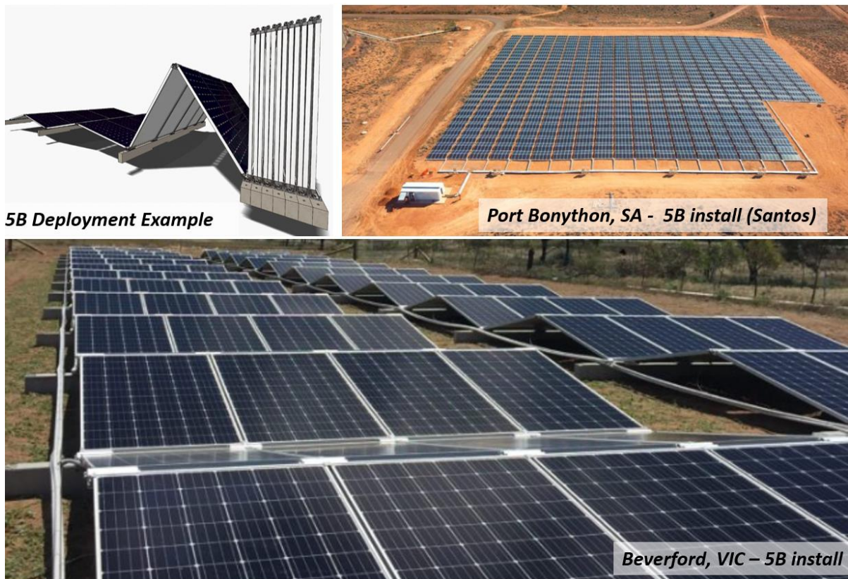
Figure 14. The 5B solar PV design. Clockwise from top-left: 5B modules are pre-assembled for rapid deployment and installation; 5B solar PV system recently installed at Port Bonython, SA, and; a previously installed 5B solar PV system in Victoria. Images obtained from 5B website: https://5b.com.au/
