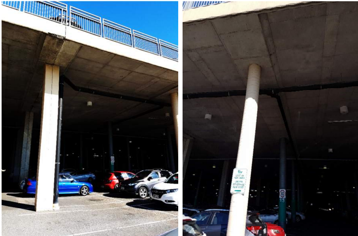
Photo 4 – Example of roof car park drainage system
