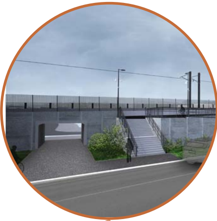
ON RAMP AND UNDERPASS
