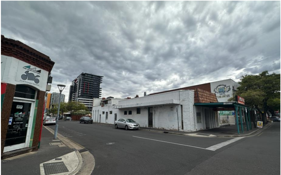
Figure 2: Subject Site viewed from intersection of Gouger and Oakley Streets
