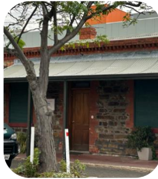
Bluestone with sand coloured pointing
