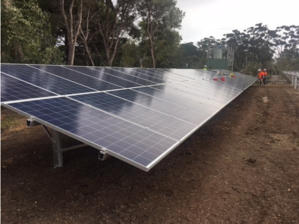
Figure 4: Typical Ground-Mounted Solar Panel Layout
