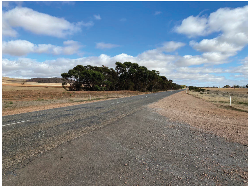
Figure 8 - Adequate sight distance to the north along Worlds End Highway (from Schulz Road)
