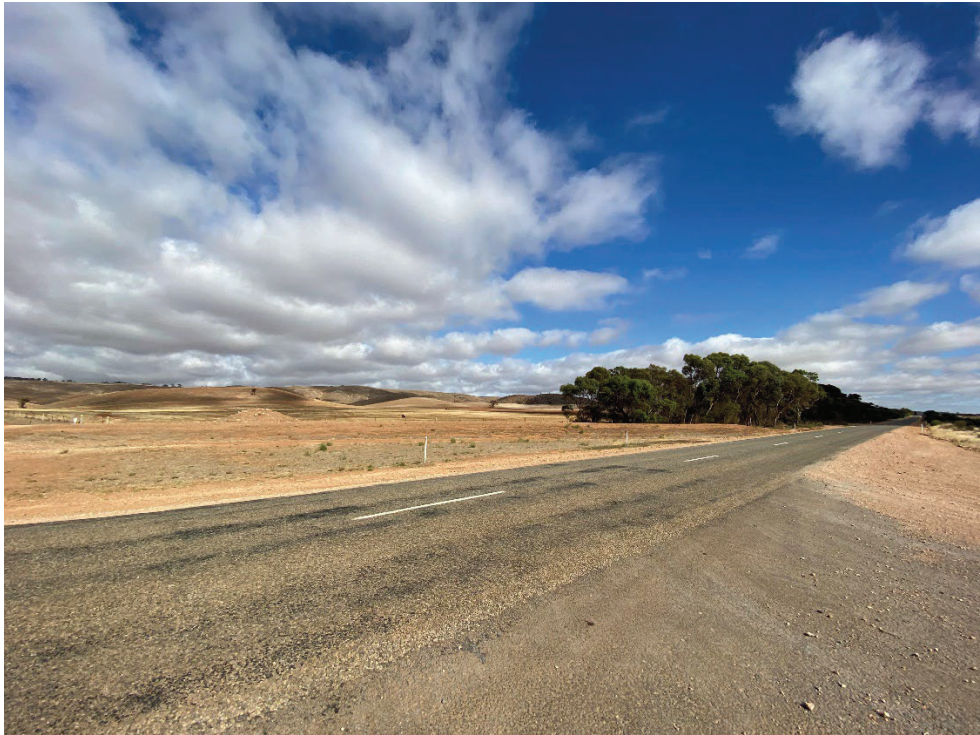
Figure 7 - Adequate sight distance to the north along Worlds End Highway (from Emmaus Road)
