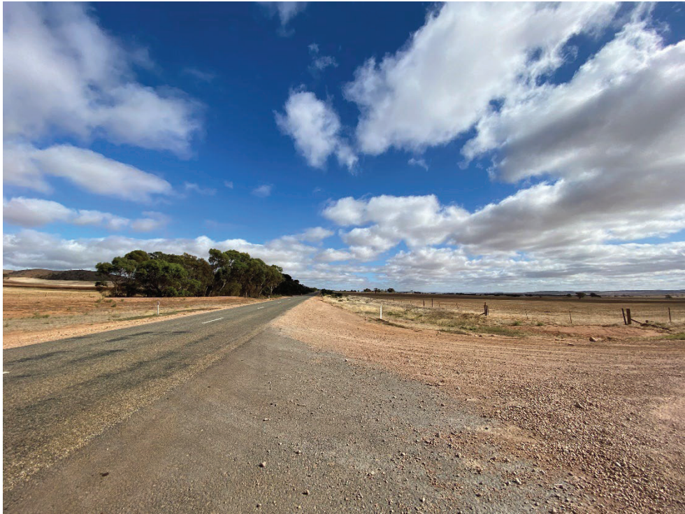
Figure 6 - Adequate sight distance to the north along Worlds End Highway (from Emmaus Road)
