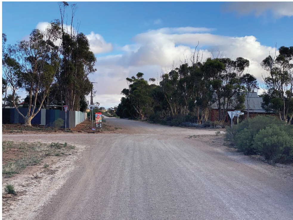
Figure 5 - Restricted corner radius at intersection of Plains Road/Australia Plains (Emmaus) Road
