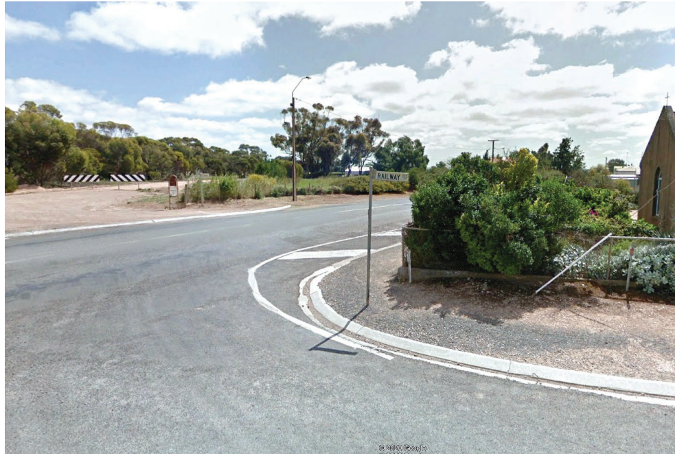
Figure 10 - Restricted sight distance to the north along Worlds End Highway (from Railway Terrace)
