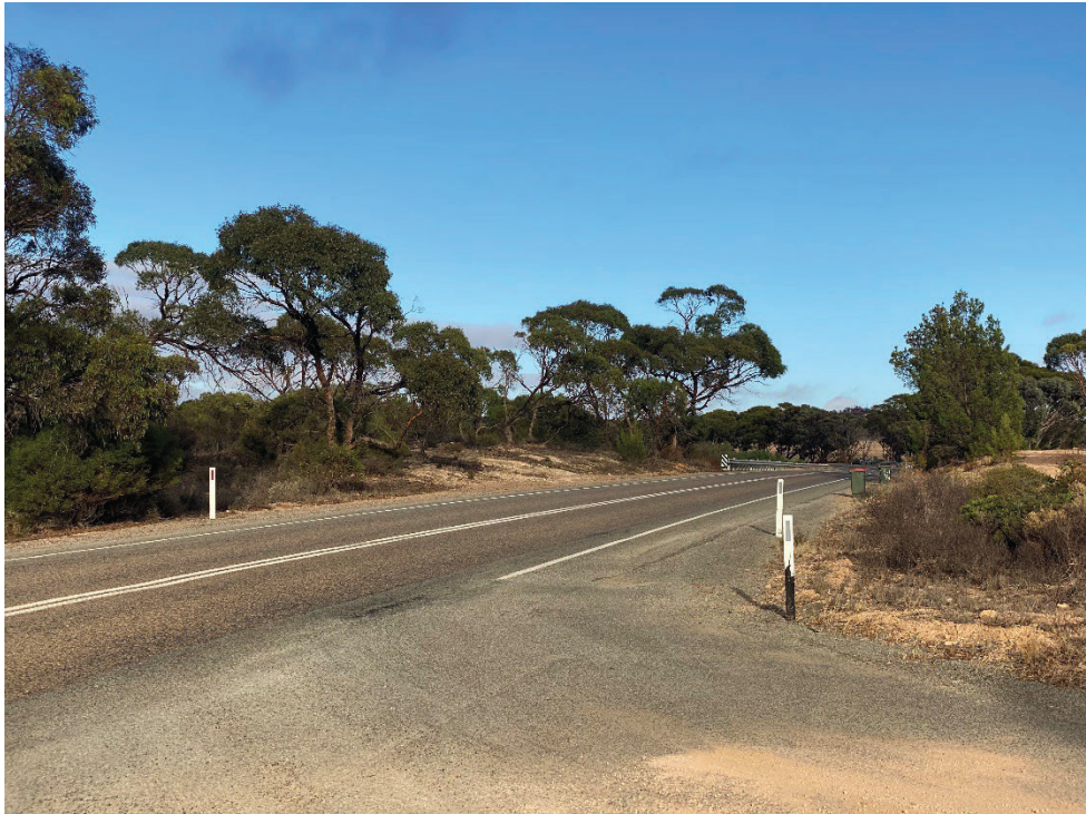
Figure 3 - Restricted sight distance to the west along Thiele Highway (from Plains Road)
