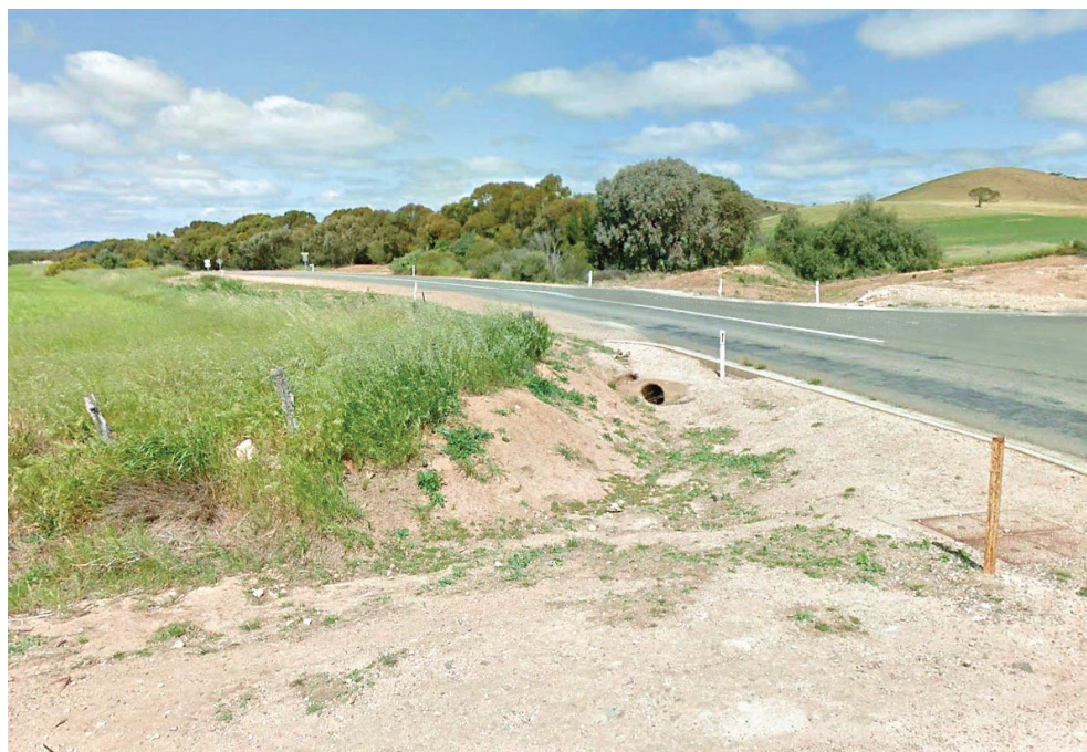
Figure 11 - Restricted sight distance to the south along Worlds End Highway (from Railway Terrace)
