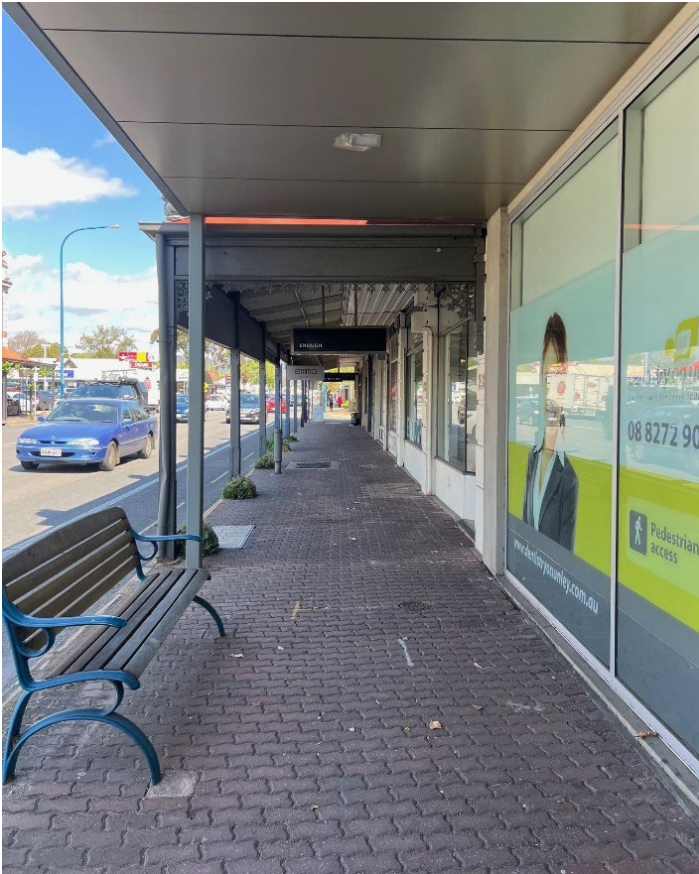
Figure 6 – Southern building footpath and verandah features
