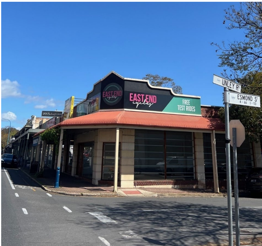
Figure 1 - Existing built form
