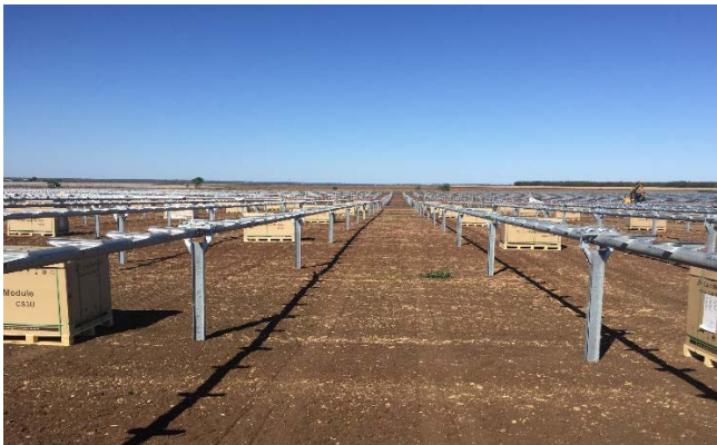
Photographs of construction and installation of single axis photovoltaic panels at RES' Emerald Solar Farm in Queensland.
