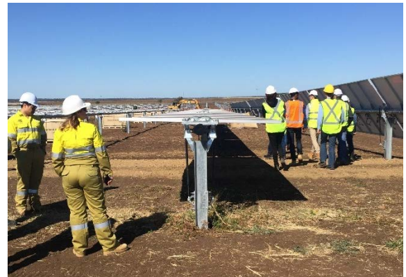
Photographs of construction and installation of single axis photovoltaic panels at RES' Emerald Solar Farm in Queensland.
