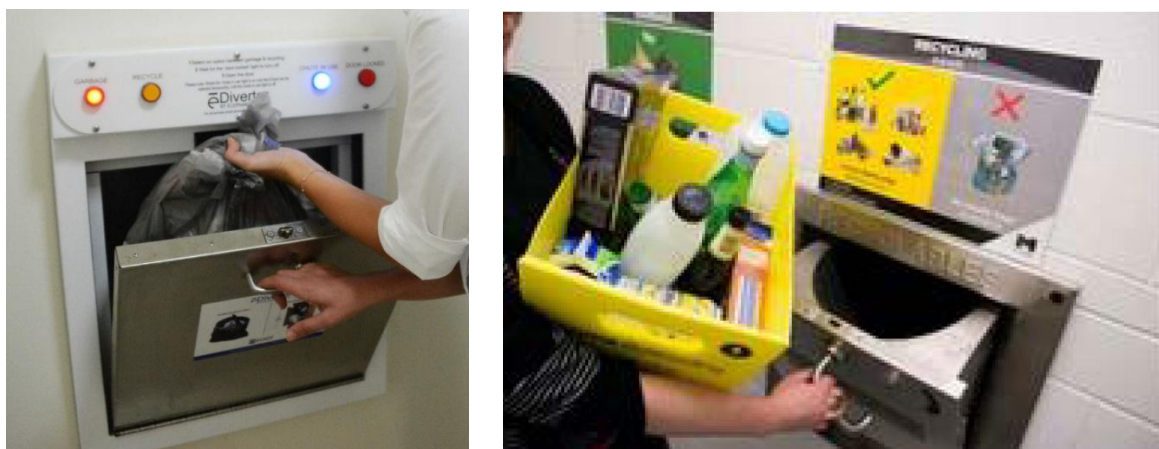
Figure 5-4 Example chute disposal access points
