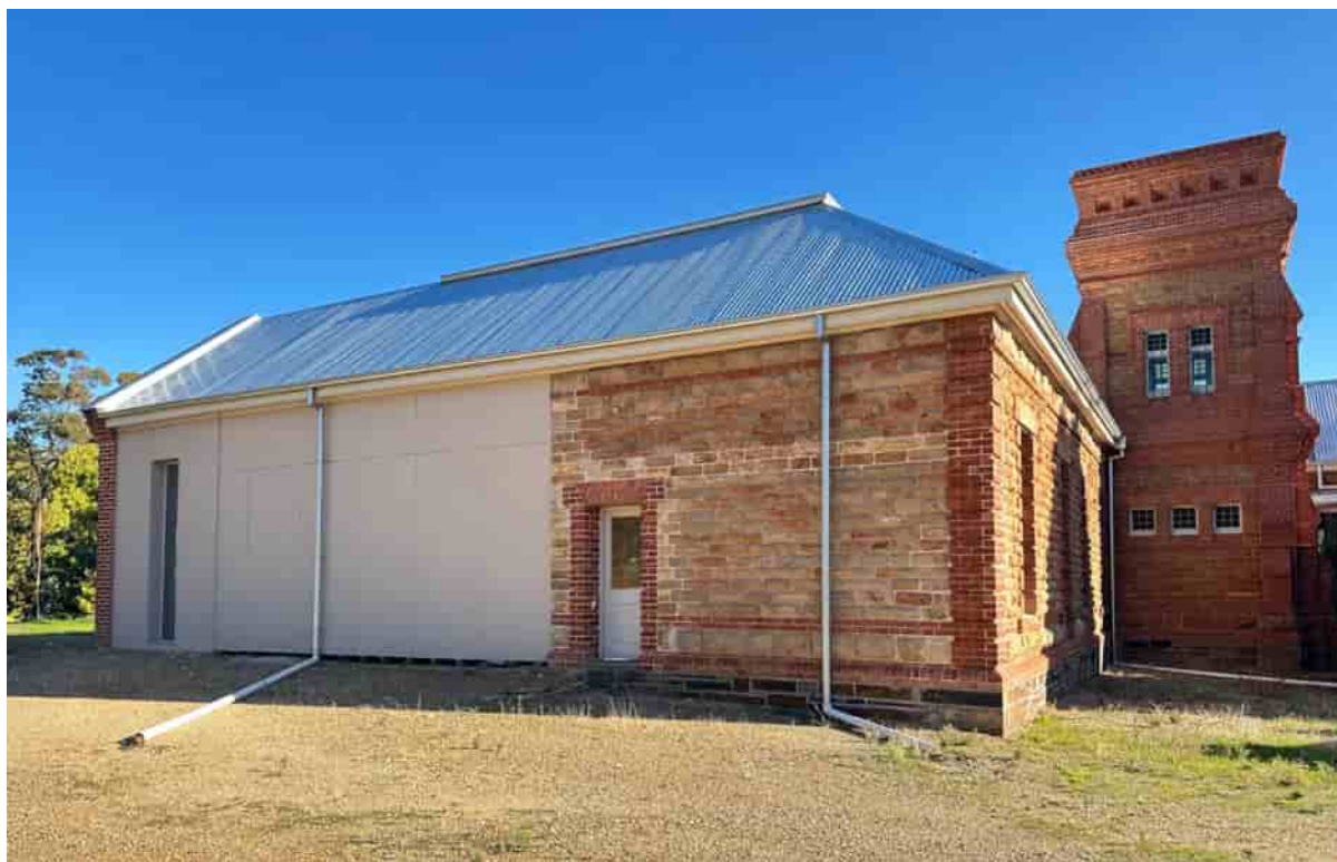
Figure 10: Eastern view of the south wing and tower, 2025 Source: Hosking Willis Architecture
