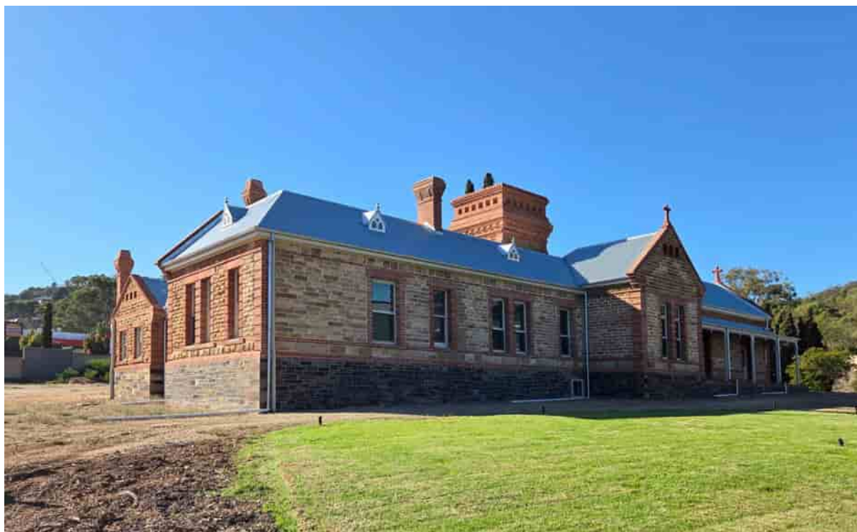
Figure 8: North-west view, 2025 Source: Hosking Willis Architecture
