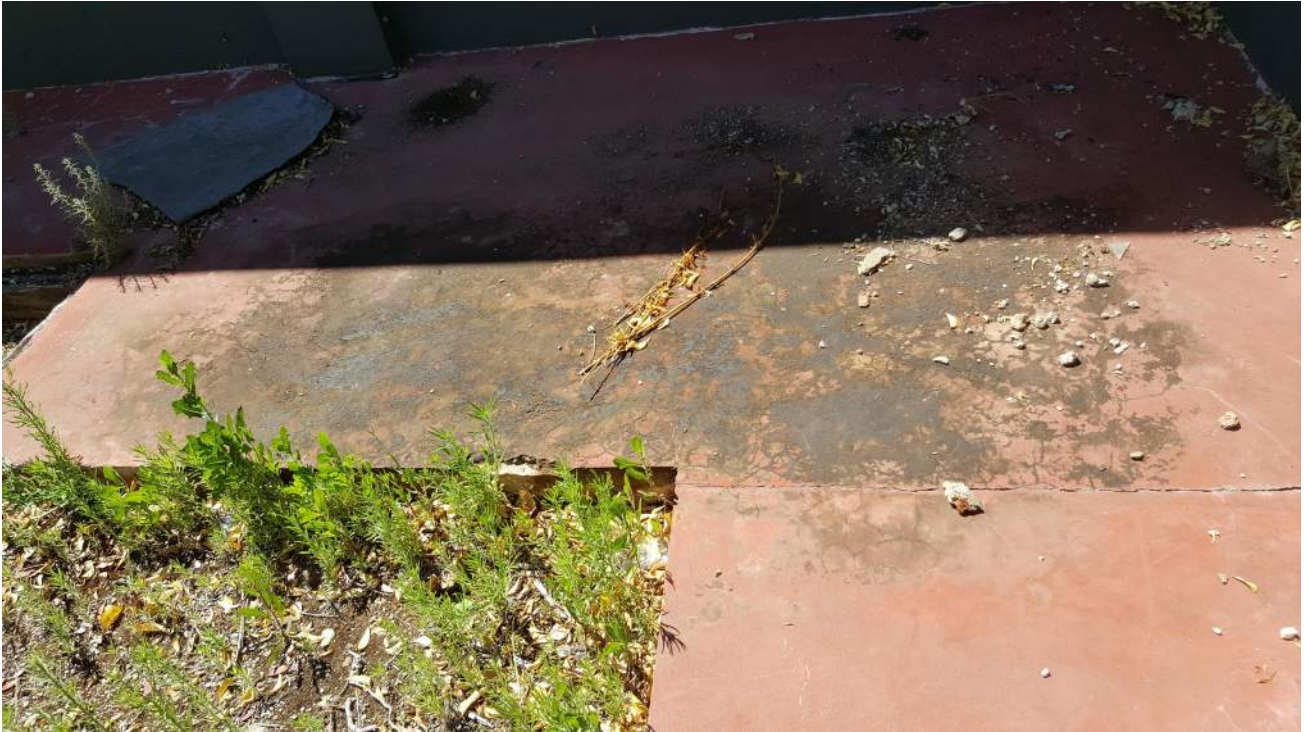
Photograph 07: View of Staining on concrete surface in north eastern corner of the site.
