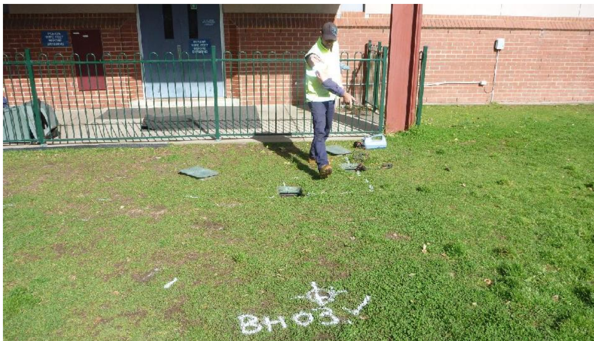
Photograph 3: Borehole BH03 location, eastern side of the Veritas Building. Photograph taken facing west.
