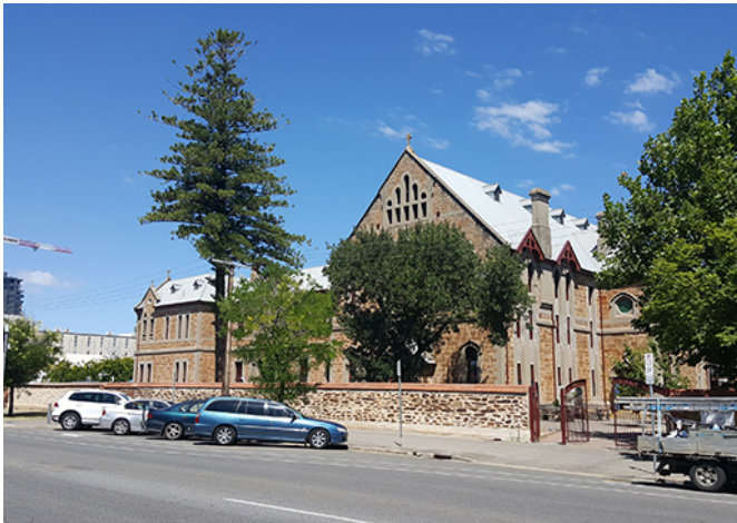
Image 1: Boylan Building, wall and main school entry gate
