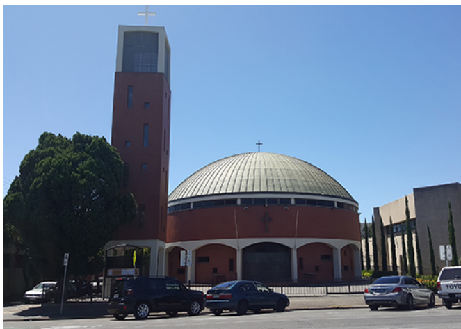
Image 7: Greek Orthodox church opposite site on Franklin Street (state heritage place)
