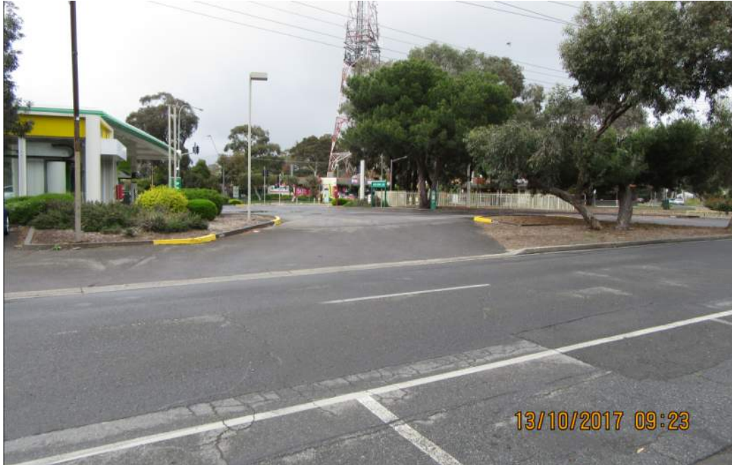
PHOTO 9: DRIVEWAY INGRESS FROM SHEOAK ROAD
