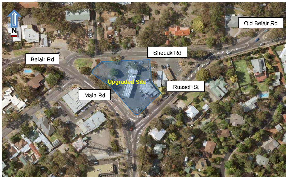
Figure 1 - Site Location at Belair (Source: maps.sa.gov, 2016)
