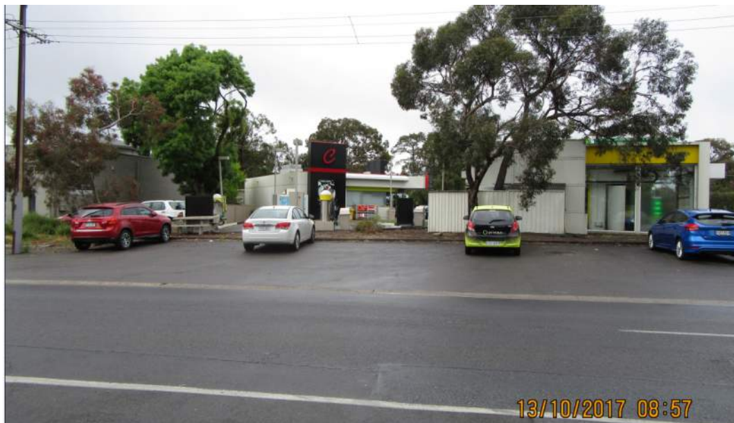
PHOTO 4: ON-STREET PARKING AREA ON SHEOAK ROAD
