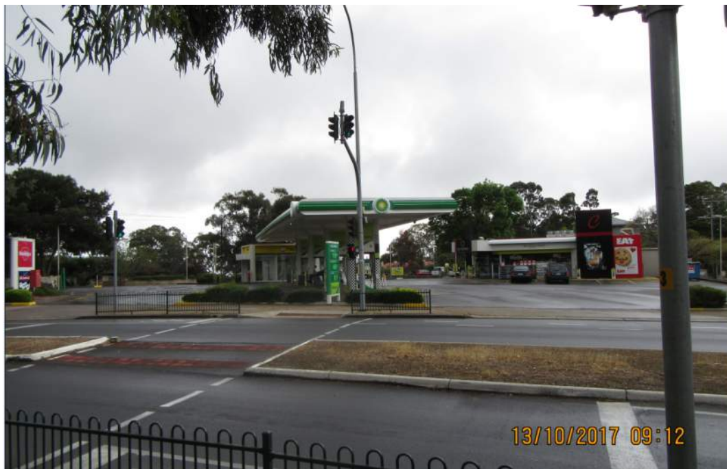
PHOTO 6: OTR BELAIR VIEWED FROM PEDESTRIAN CROSSING ON MAIN ROAD
