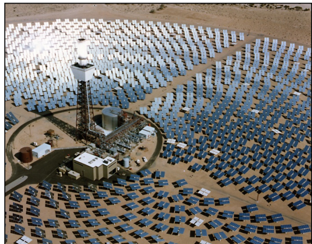
Figure 6 - An example of glare from the receiver and the collector field during normal operation
