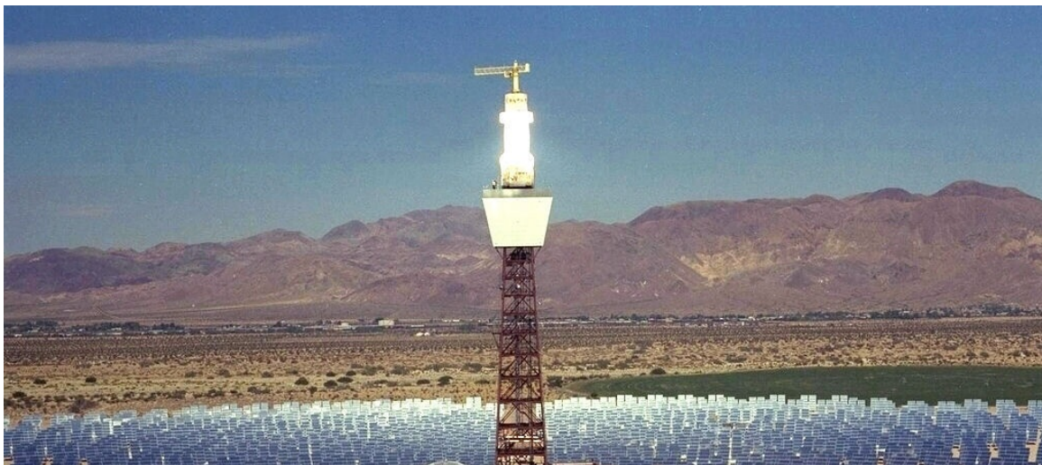
Figure 19 – Solar Two receiver during full power operation (Barstow, CA, U.S.A)
