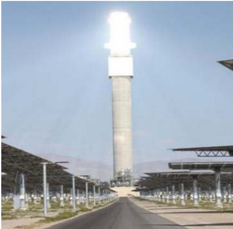
Figure 5-1 Crescent Dunes Tower
