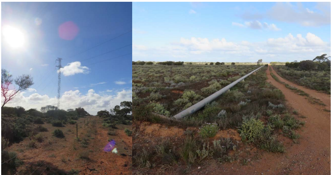
Figure 4-6 Existing transmission line and water pipeline
