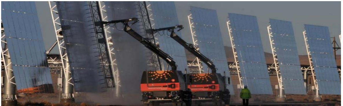
Figure 2-9 Example of cleaning
