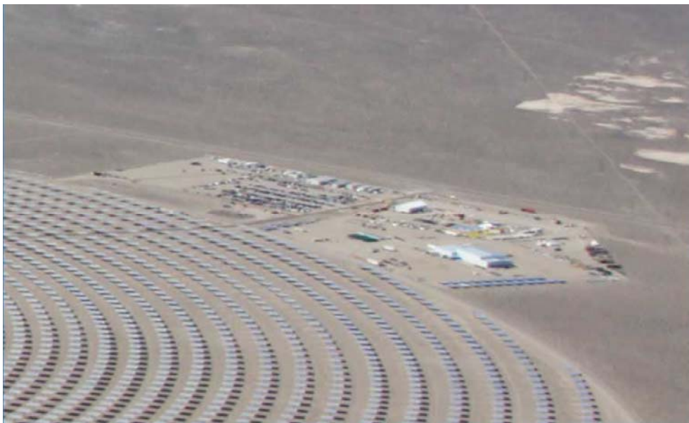
Figure 2-10 Example of construction facilities
