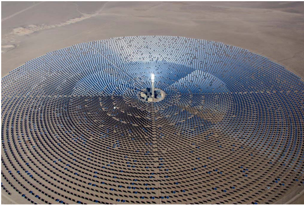
Figure 2-3 Heliostat field arrangement
