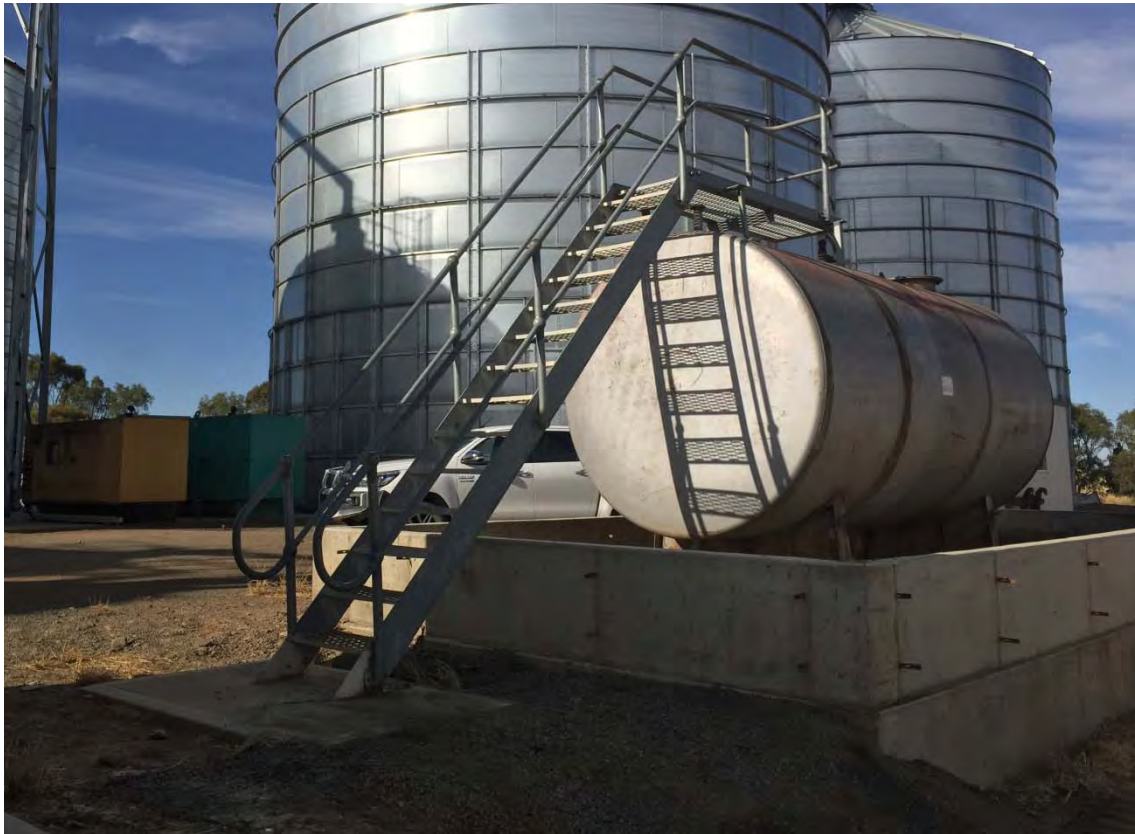
Photograph 4 – Diesel storage tank and bund
