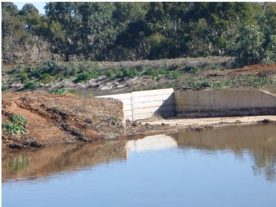
Photograph 12 – Sedimentation basin horizontal slatted weir control outlet
